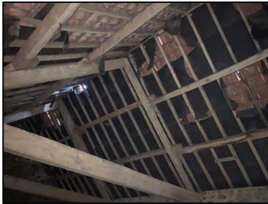
Photo 5: Bitumastic-lined roof inside building A.
