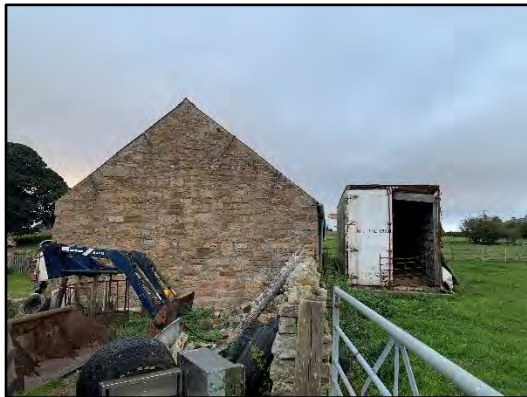
Photo 19: South gable end of building E.
