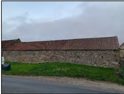
Photo 11: West aspect of Building C.
