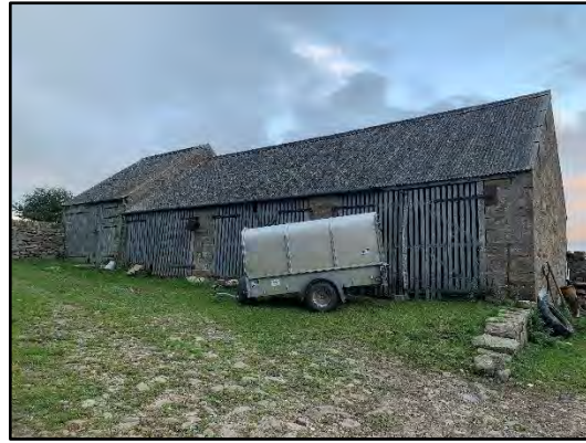
Photo 18: West aspect of building E.
