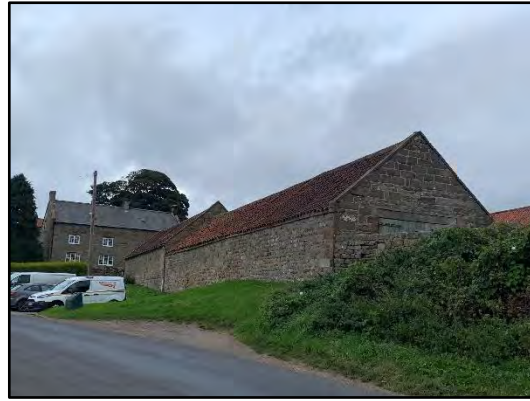
Photo 10: South-west aspect of building's C and B from the road.
