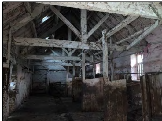
Photo 16: Inside building D.
