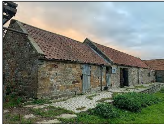
Photo 12: Western aspect of building D.
