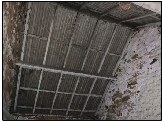
Photo 20: Corrugated roof of building E.
