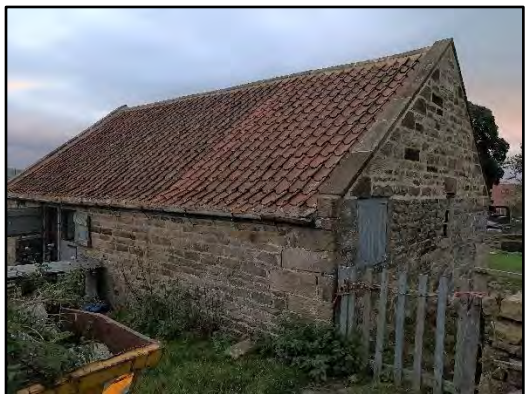
Photo 21: North-eastern aspect of building F.
