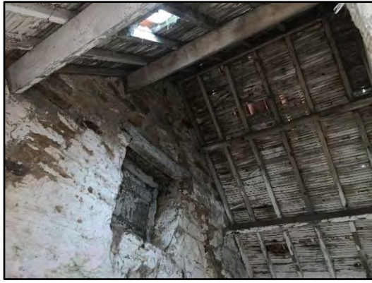
Photo 17: Lathe-lined roof in building D.
