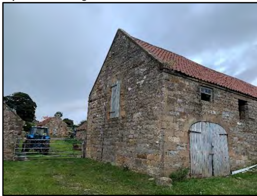
Photo 3: South-west gable end of building A.
