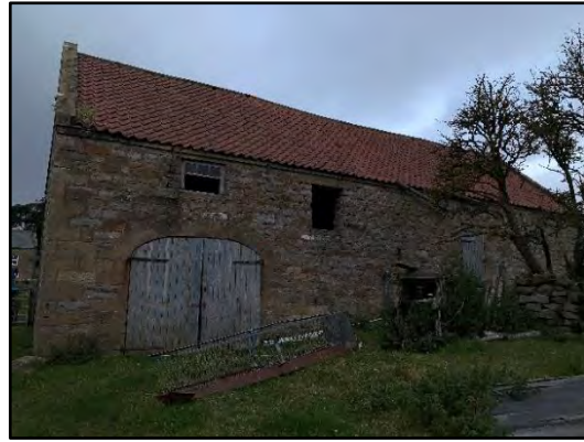
Photo 2: Southern aspect of building A.
