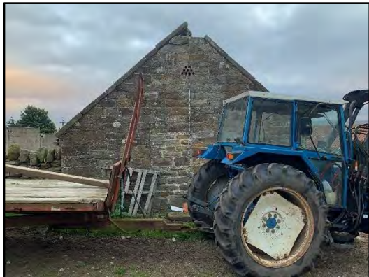
Photo 13: North gable end of building D.
