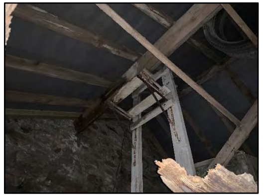
Photo 24: Bitumastic-lined roof of building F.
