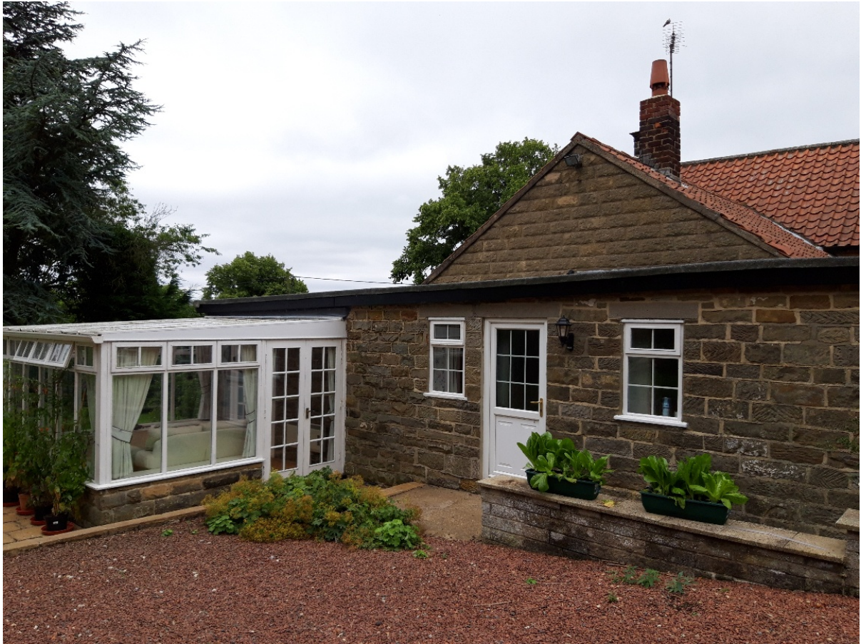
This photo shows the rear elevation of the property, including the existing sunroom to be replaced.
