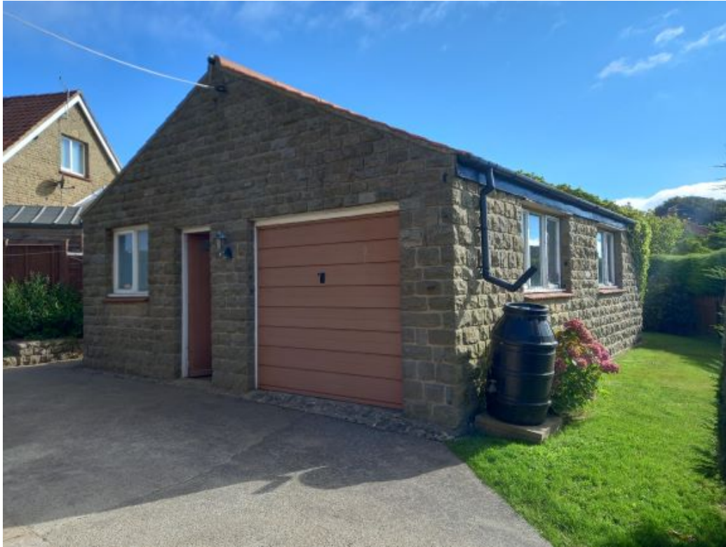
Photograph of garage building taken from the driveway. It is constructed of stone under a clay tile roof. The gable facing the side elevation of the house is characterised by a garage door, personnel door and window, with two further windows in the side elevation facing the roadside boundary.
