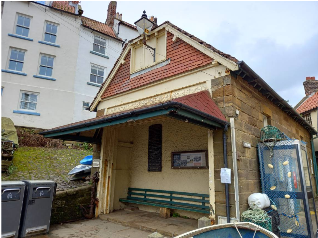
This photograph shows the shelter and canopy of the Public Conveniences.
