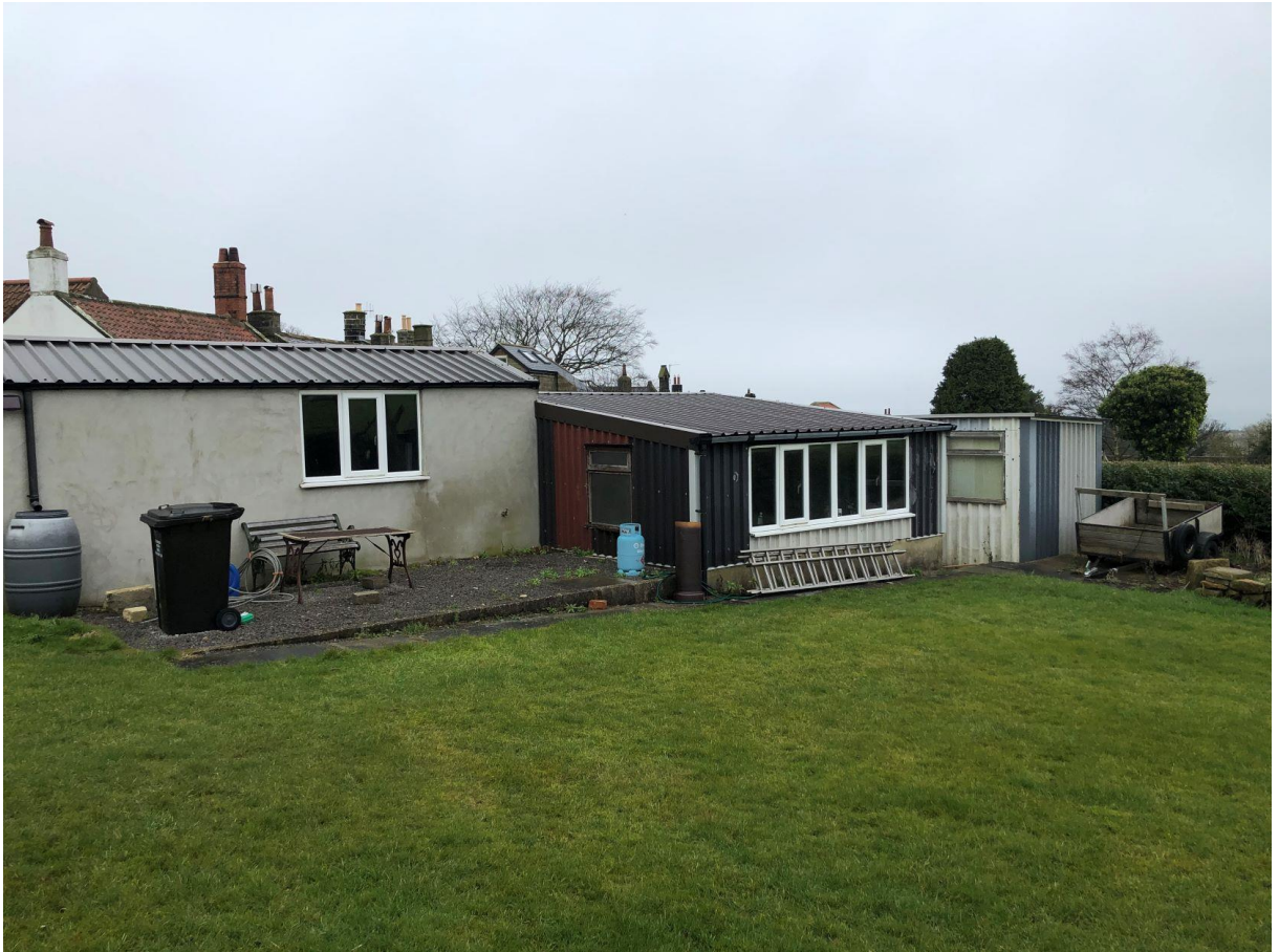
Photograph 3 Range of utility buildings with No.4 to the rear
