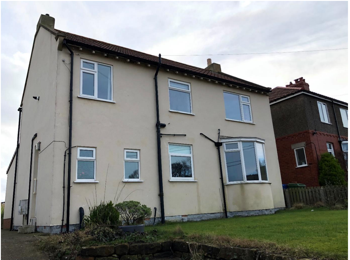
Photograph 1 Front (north) road side elevation
