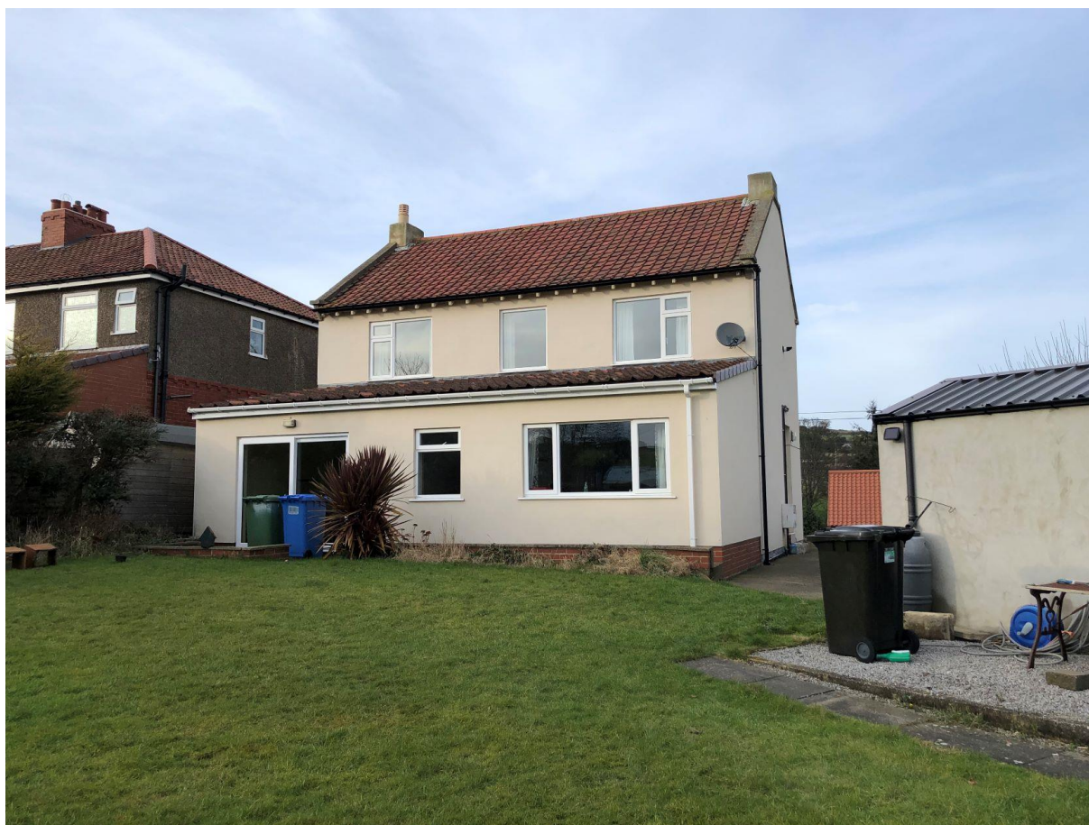
Photograph 4 Rear viewed from south-east
