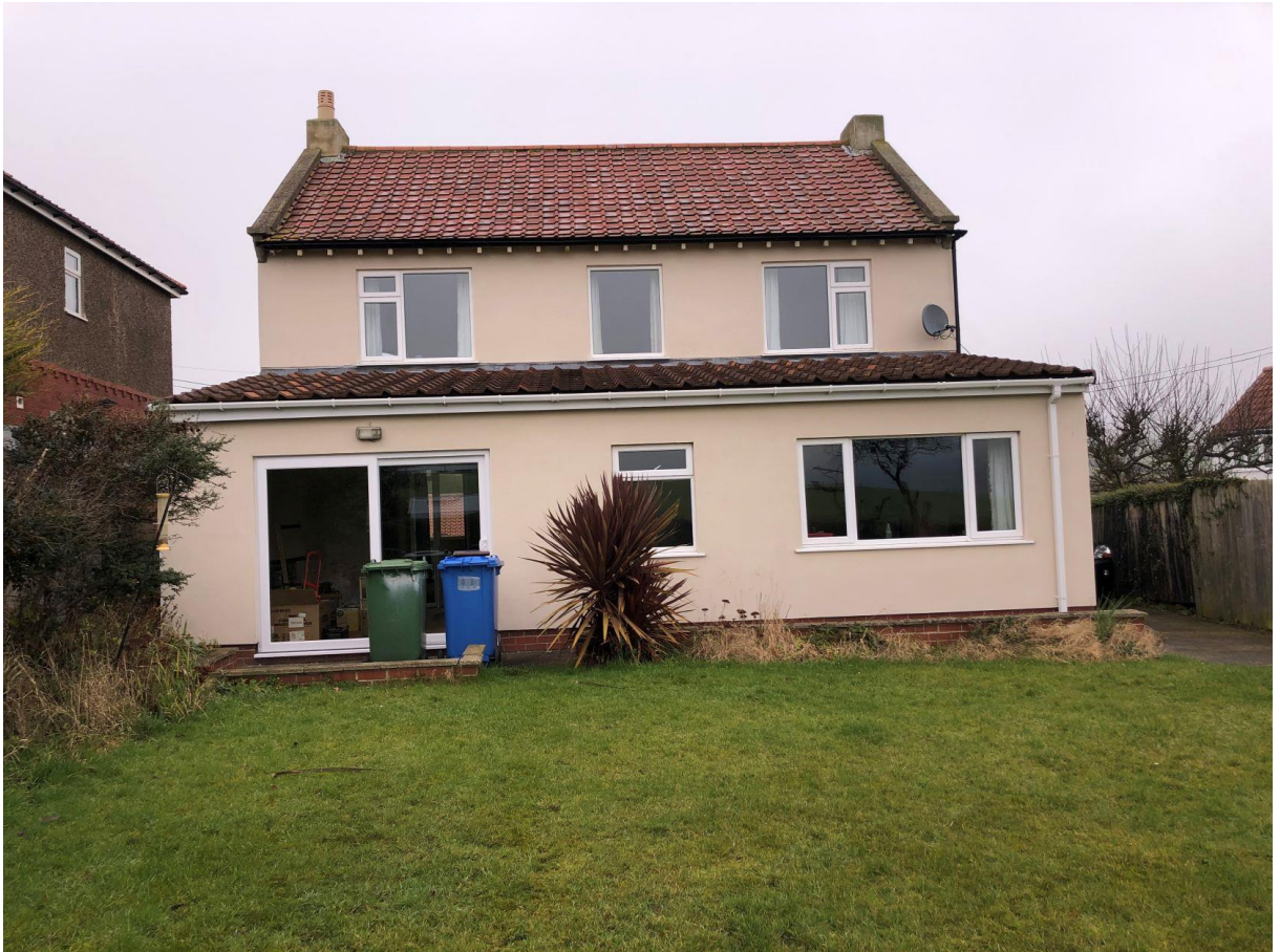
Photograph 2 Rear (south) elevation
