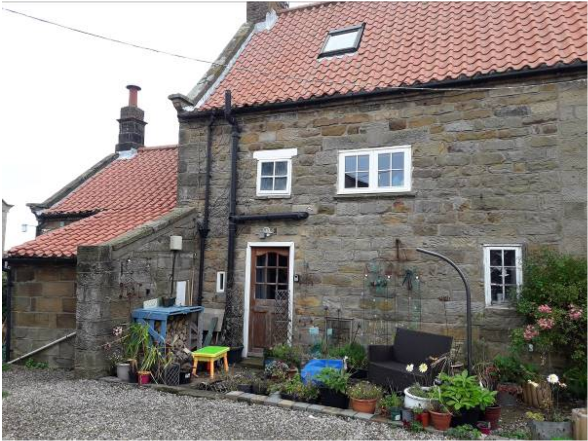
Photo showing rear elevation of Manor Farm Cottage, Newholm.
