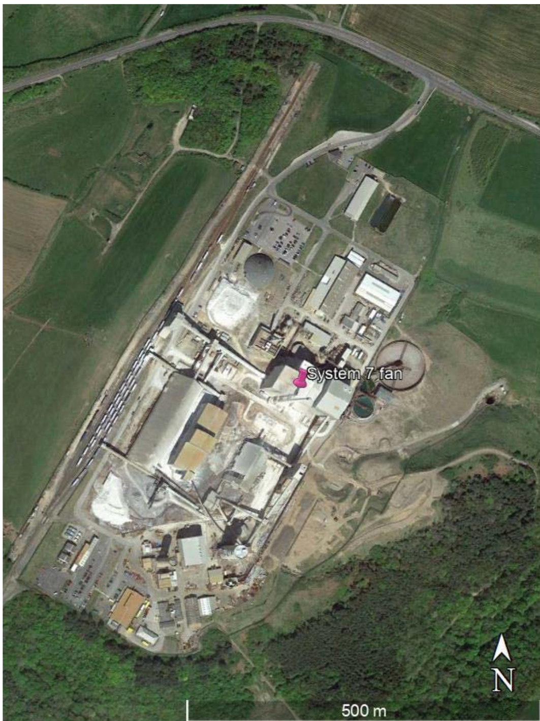
Figure 4.13 Location of System 7 fan
