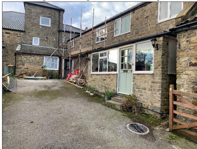
Figure 7 – Existing Extension at The Cottage
