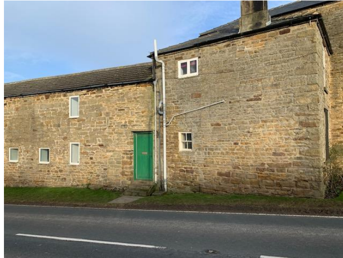
Figure 4 – Existing Door and Small Window to be replaced
