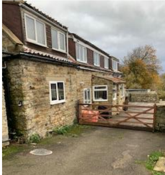
Figure 8 - Existing Dormer Extensions
