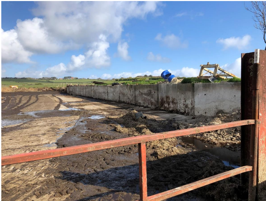
Fig 4. – Site of manure store and proposed roof/structure over.
