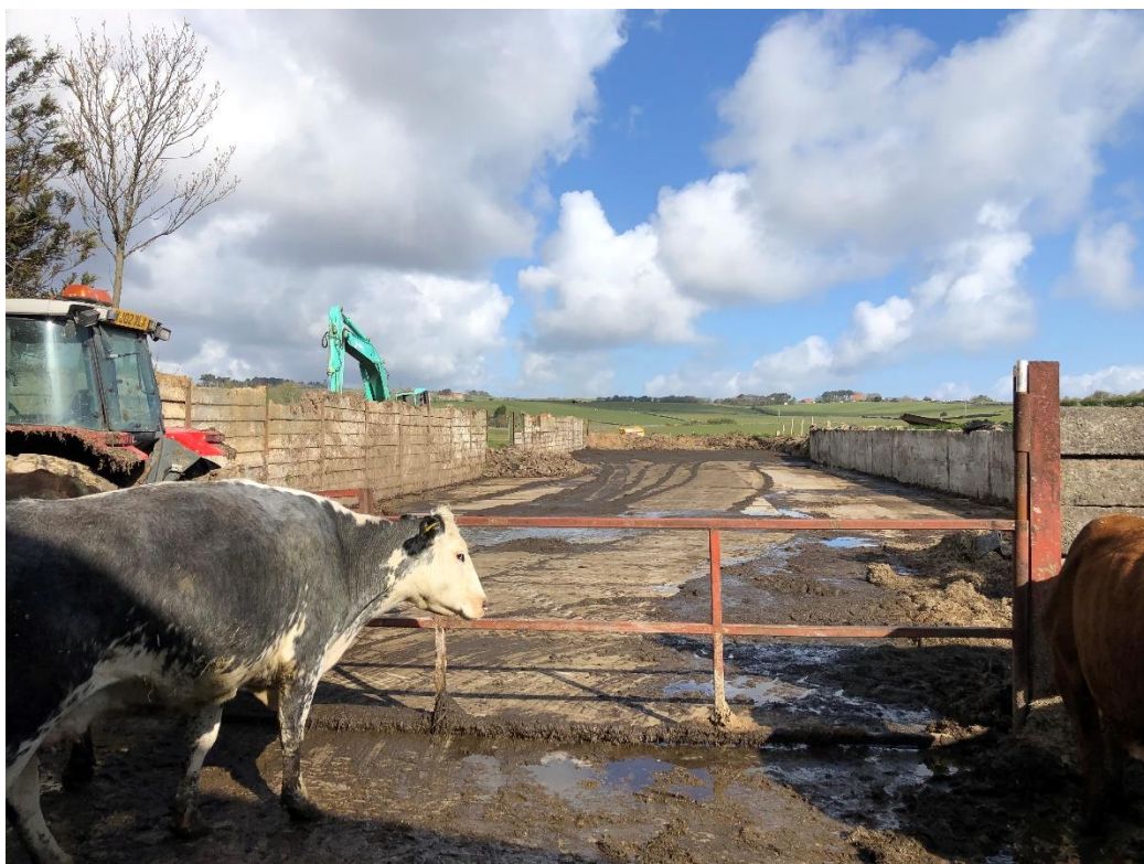
Fig 5. – Proposed site for roof structure.
