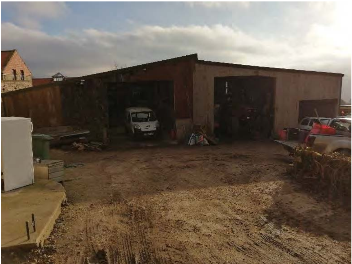
Building 1 after wall cladding carried out and open end section walled in to left of picture
