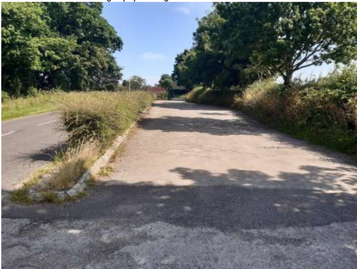
Southern end of layby looking north
