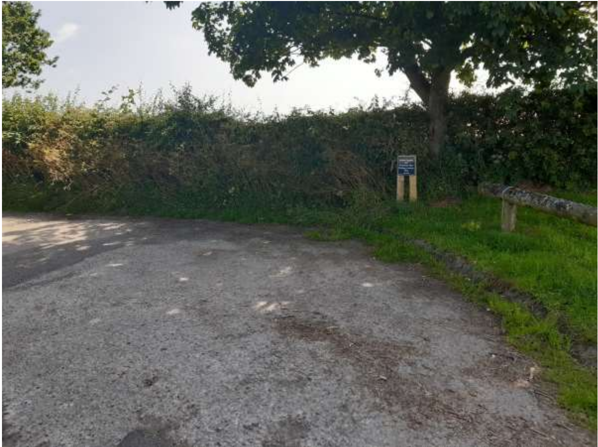
Southern end of the existing layby looking east
