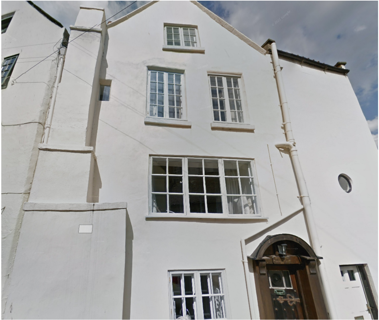
Front elevation of Fisherman's Cottage.
