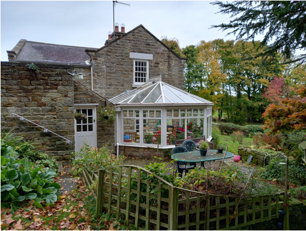
The west (side) elevation of Cawood Cottage with existing conservatory.
