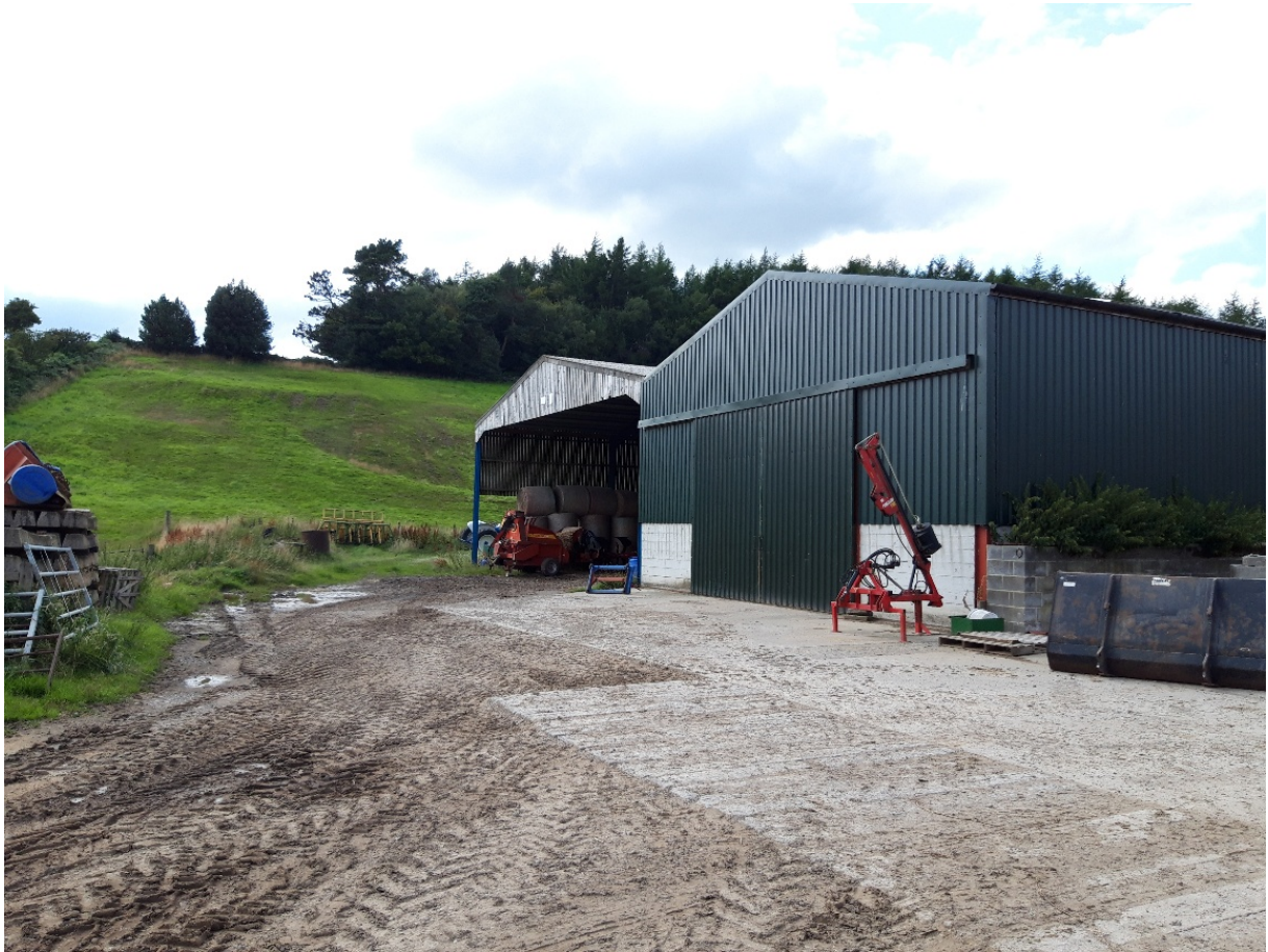
This photo shows the two existing sheds, alongside which the proposed shed will be constructed.
