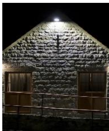
Shielded warm white lights with appropriate controls provide directed light only where and when it is needed.
