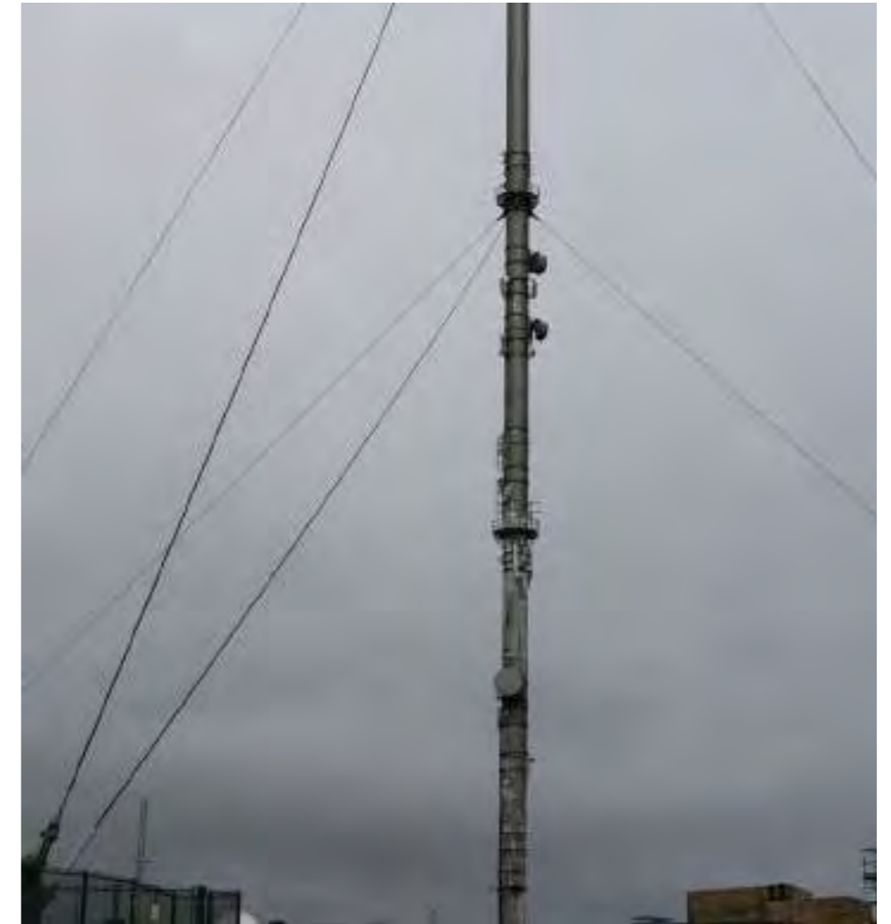
Figure 2: Image of the existing (now demolished) solid mast construction
