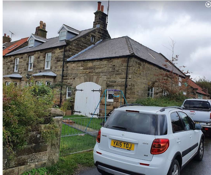
Holme Garth with adjoining former Smithy. The red roof of the earlier vernacular house can be seen at the far left.
