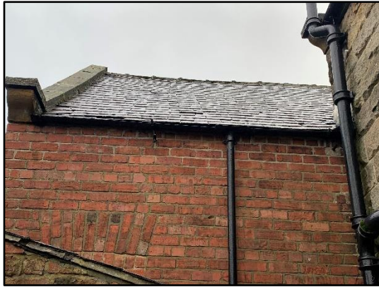
Photo 3: North-facing wall and roof.
