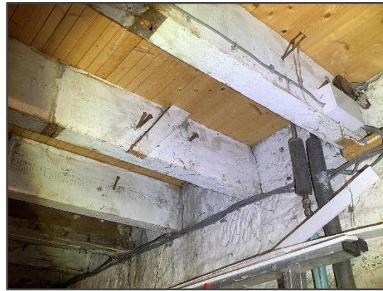
Photo 6: Ground floor boarded ceiling with timber frames.
