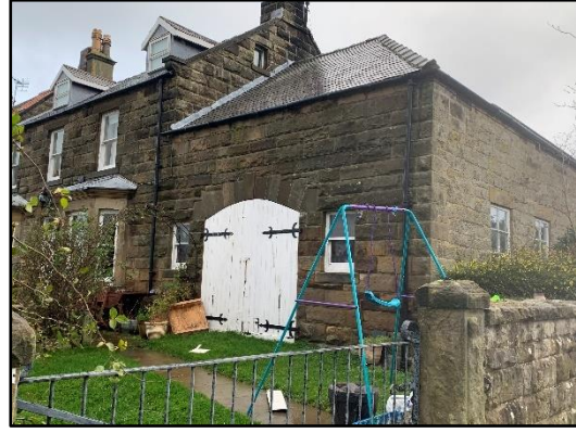
Photo 2: South-west aspect aspect of the building.
