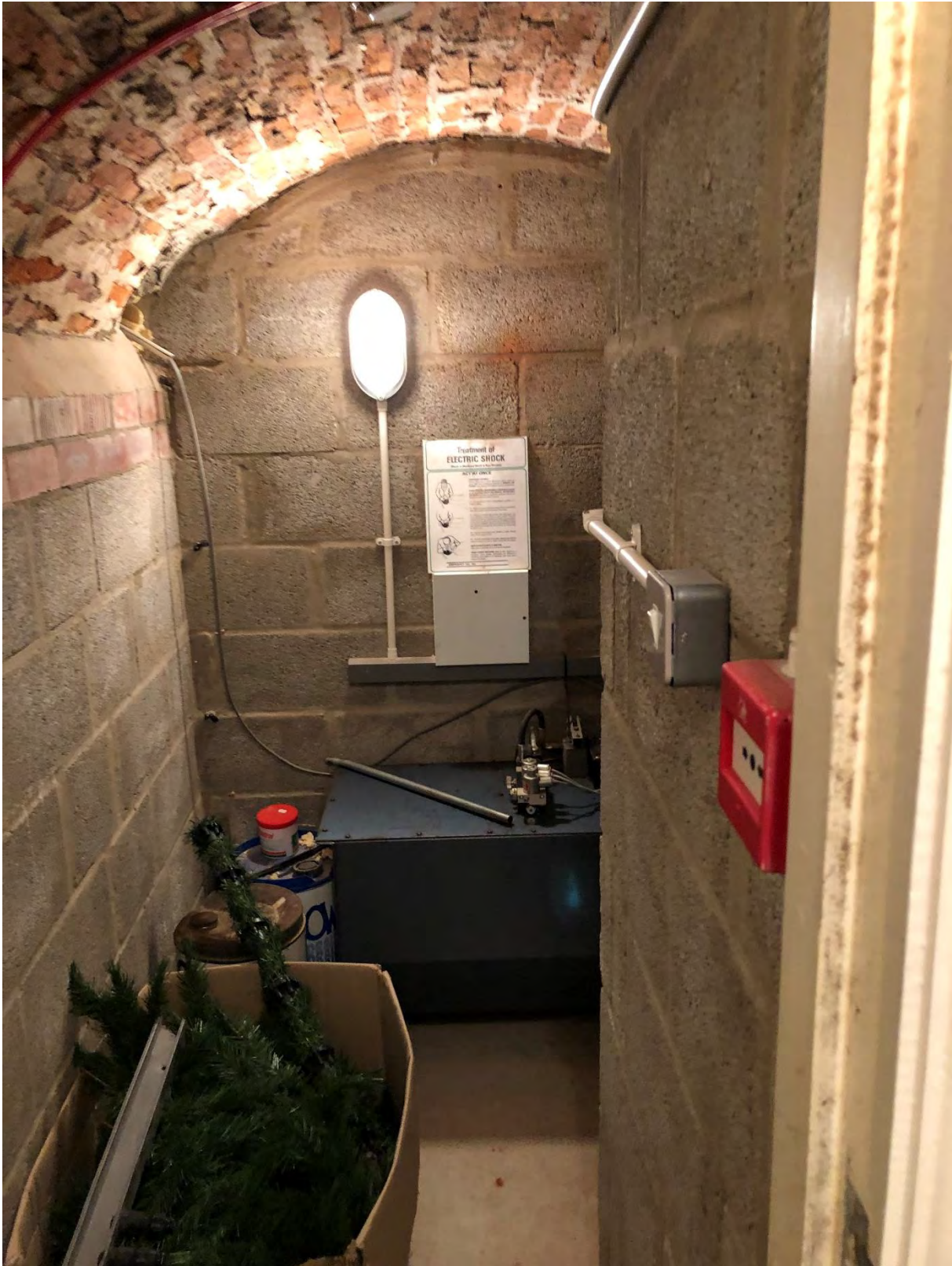
Plant room (part of brick vaulted ceiling)
