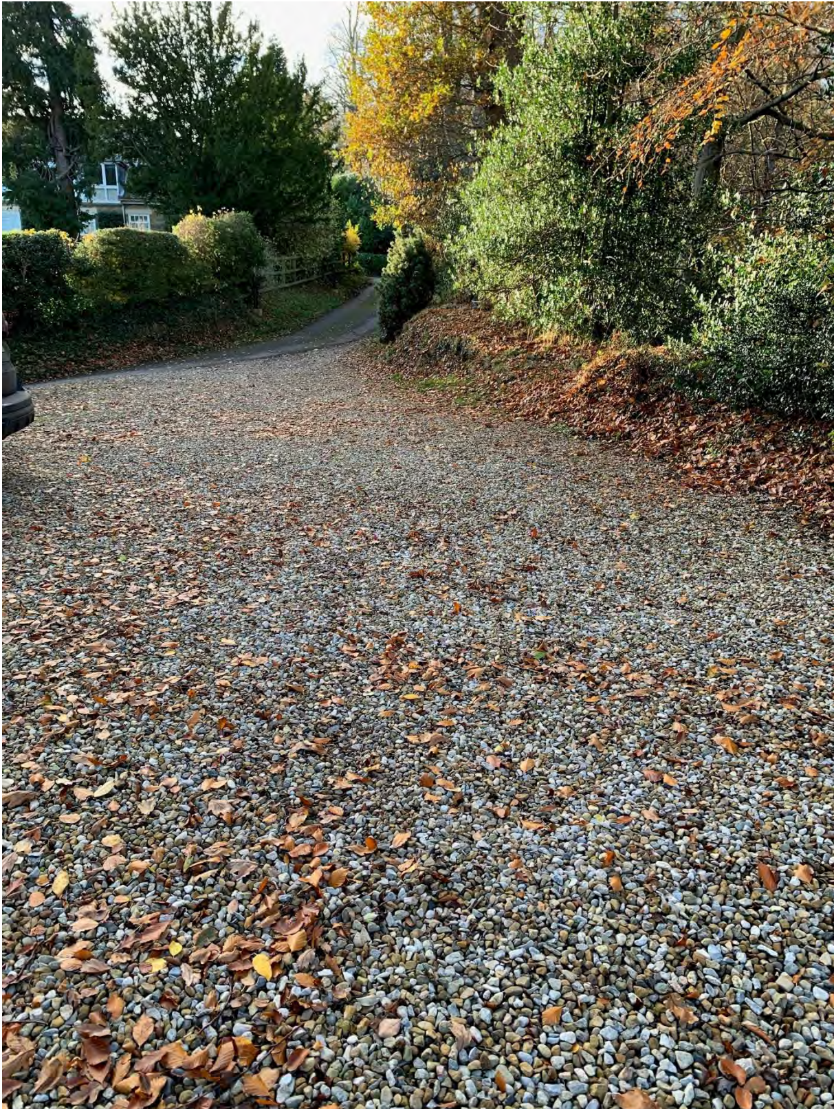
Car Park entrance with access drive on right and Woodlands Apartments behind the hedge and trees
