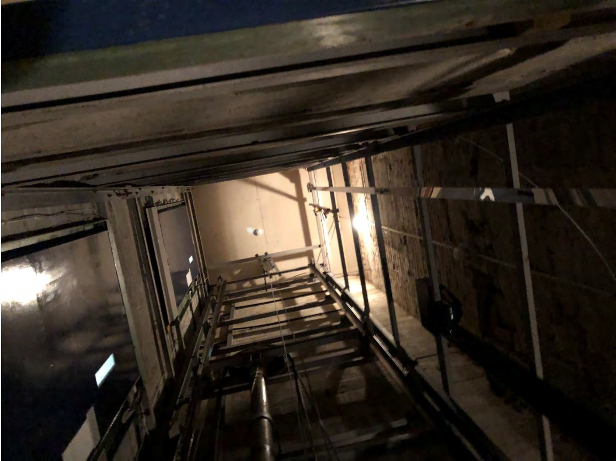
Looking up the lift shaft (doors on the left)
