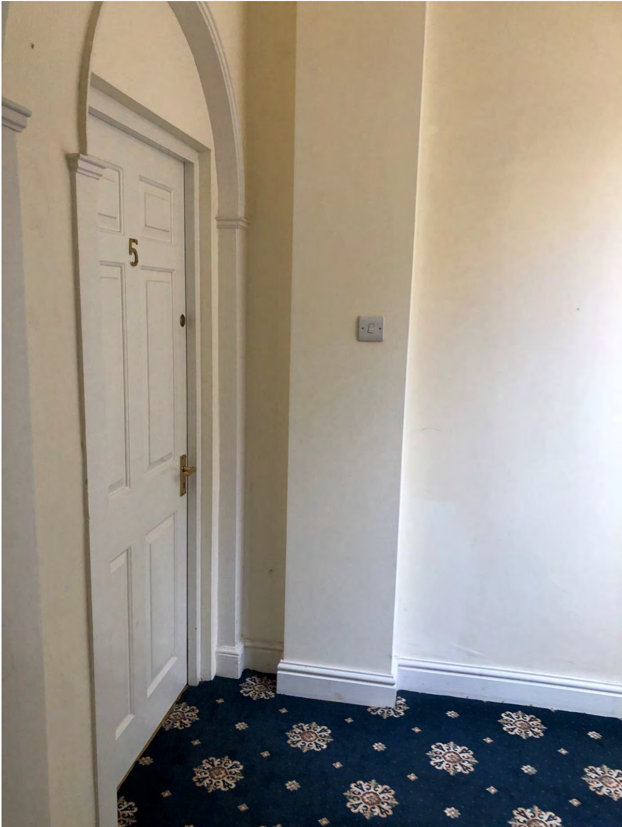
Entrance door and landing to Apartment 5
