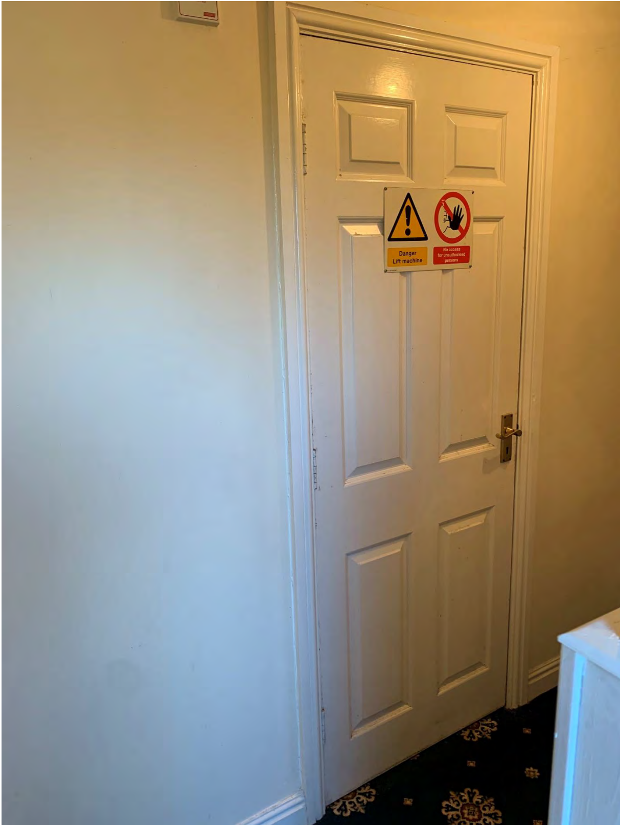
Plant room door, architraves and skirting boards (Looking towards the lift)
