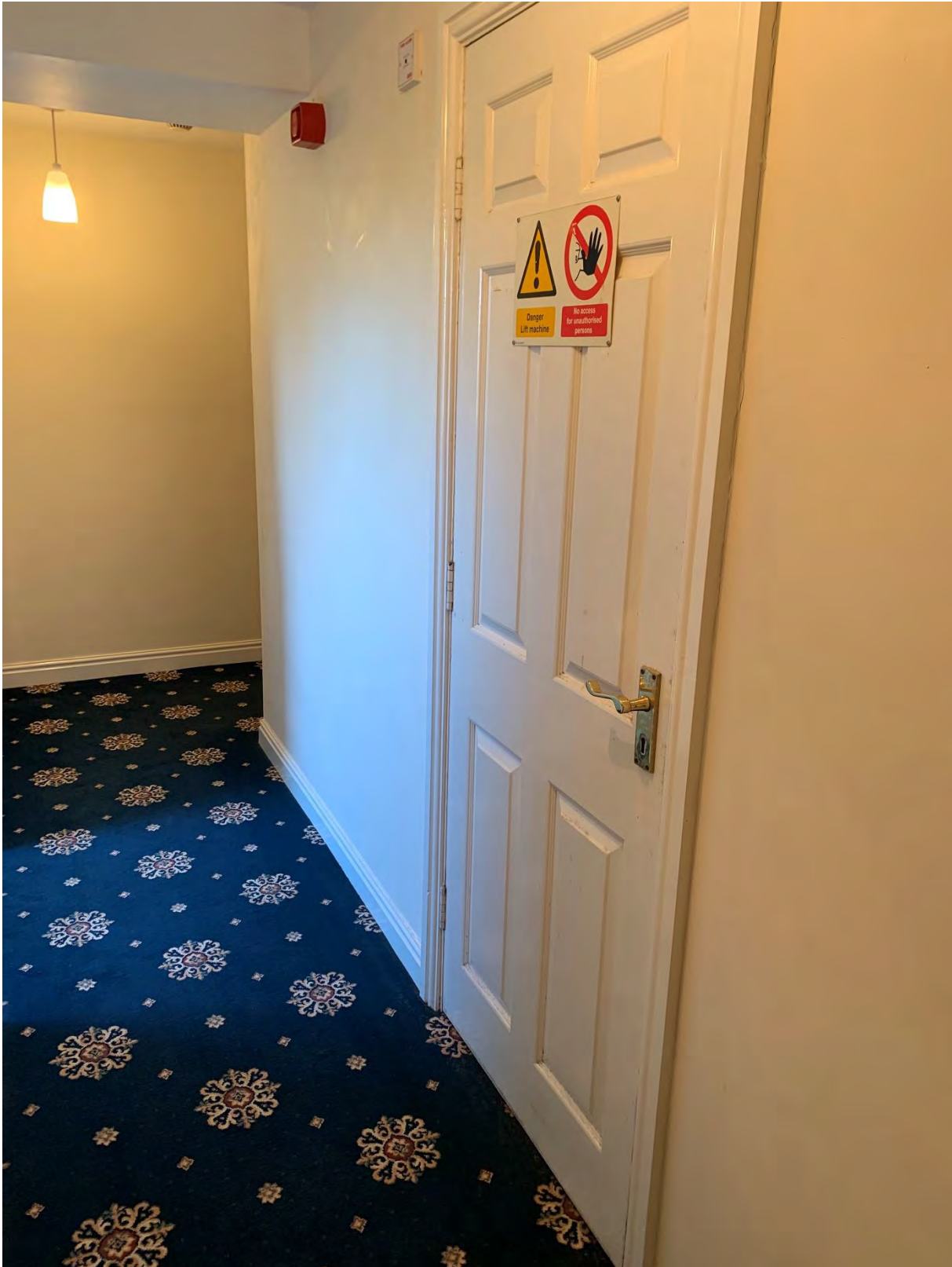
Plant room door (Looking towards corridor and access route)
