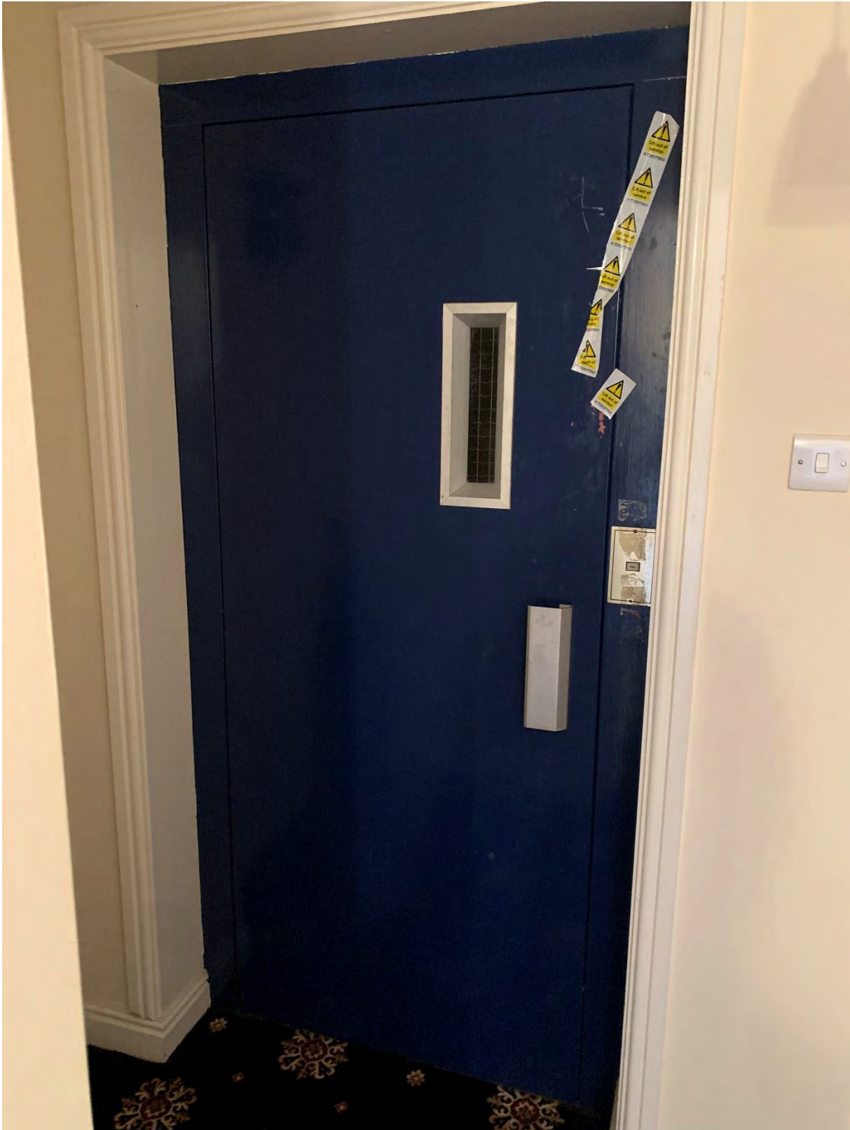
Lift door, architraves, linings and skirting boards
