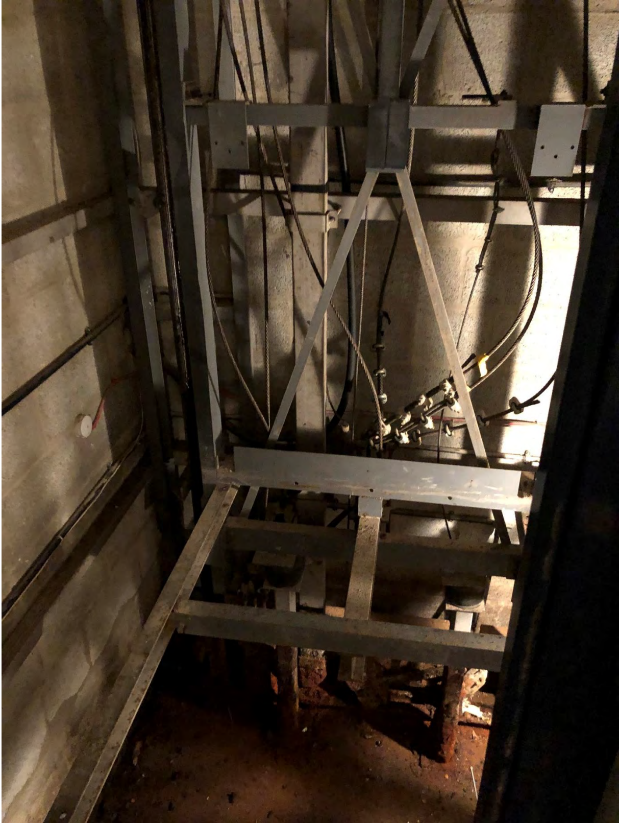
Rear wall of lift shaft (sump at bottom)
