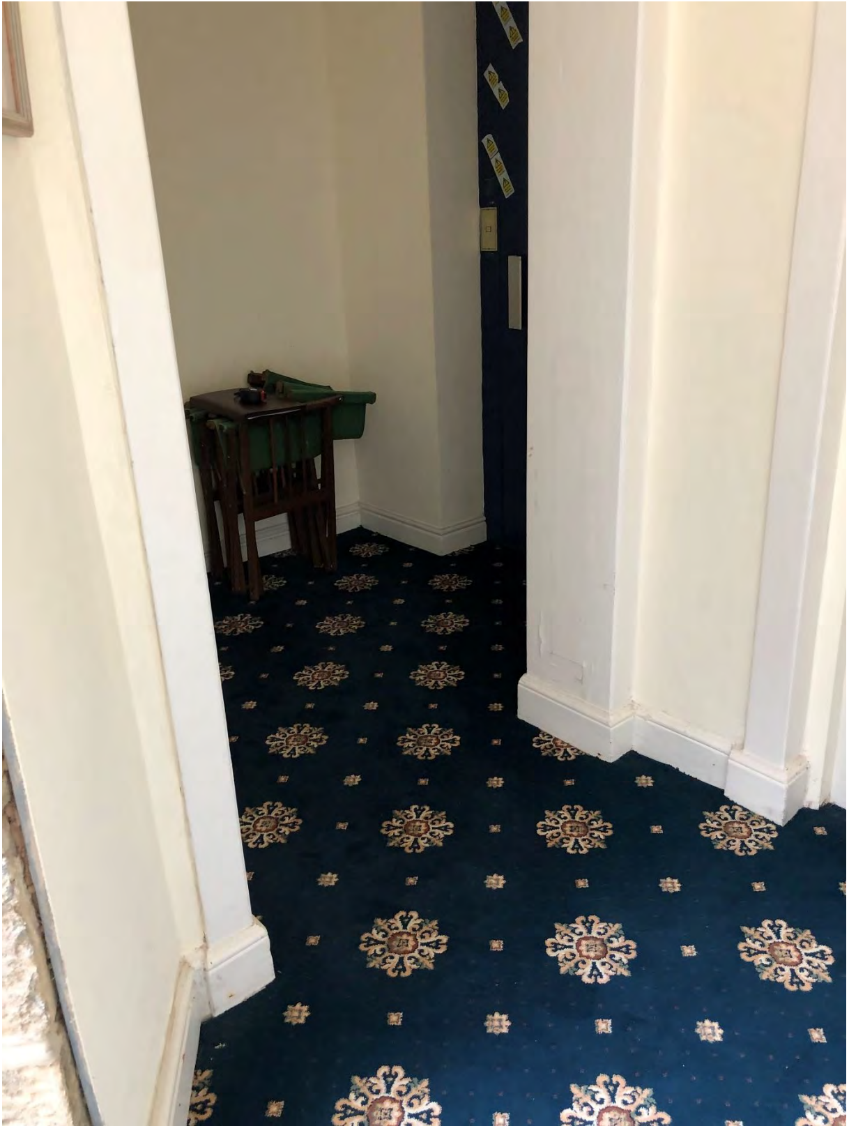
Skirting boards and timber linings to arches
