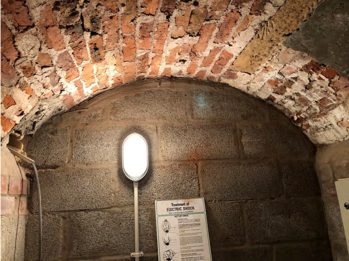
Plant room (full brick vaulted ceiling)
