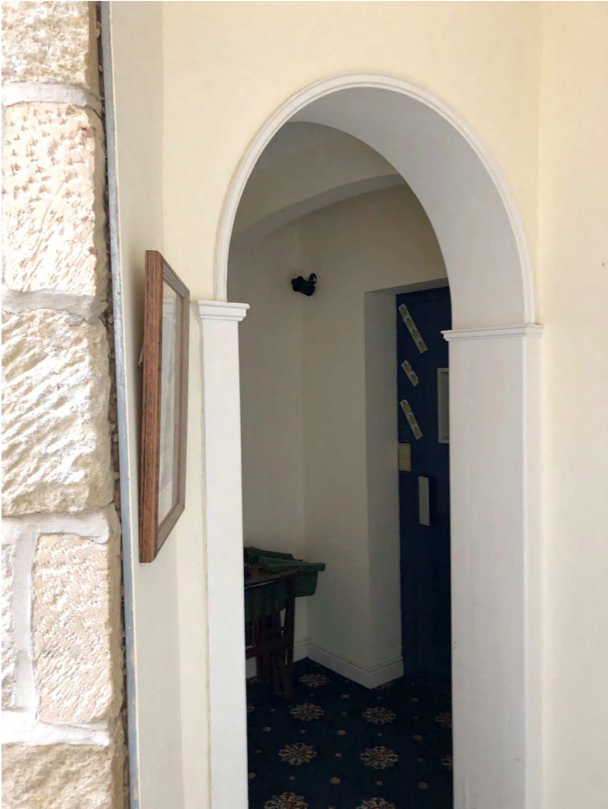
Arches and Lobby to Lift door
