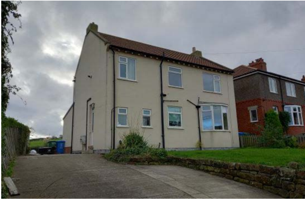
Front elevation of Glendower as seen from the pavement. The property is a detached two storey dwelling finished in cream render under a pantile roof (ridge parallel with the road). The main access door is in the side elevation and the front is characterised by a bay window at ground floor level on the right with three smaller windows to the left and three standard windows at first floor.
