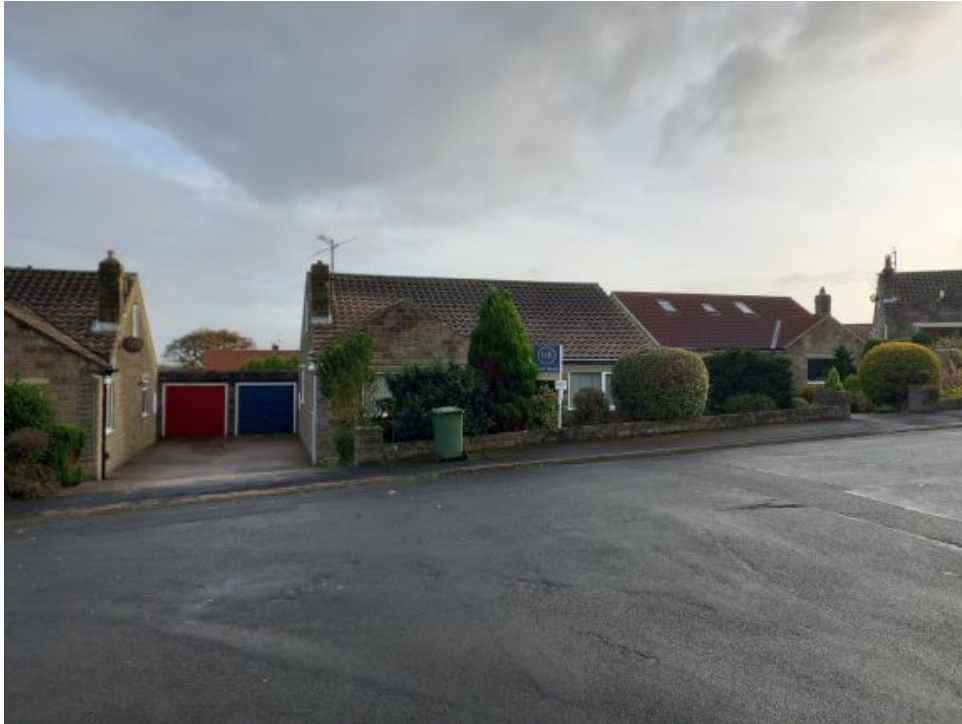
Front elevation taken from within Kingston Garth. The application property is a bungalow, central in the picture with a semi-detached flat roof garage with blue door to the left. The front elevation is partially obscured by large garden shrubs.
