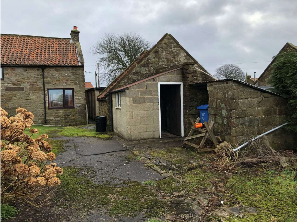
Photograph 3 Rear/West Elevation showing stone and clock lean to buildings
