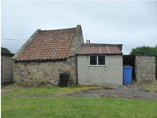
Outbuildings 1,2 and 3 (from LHS)
