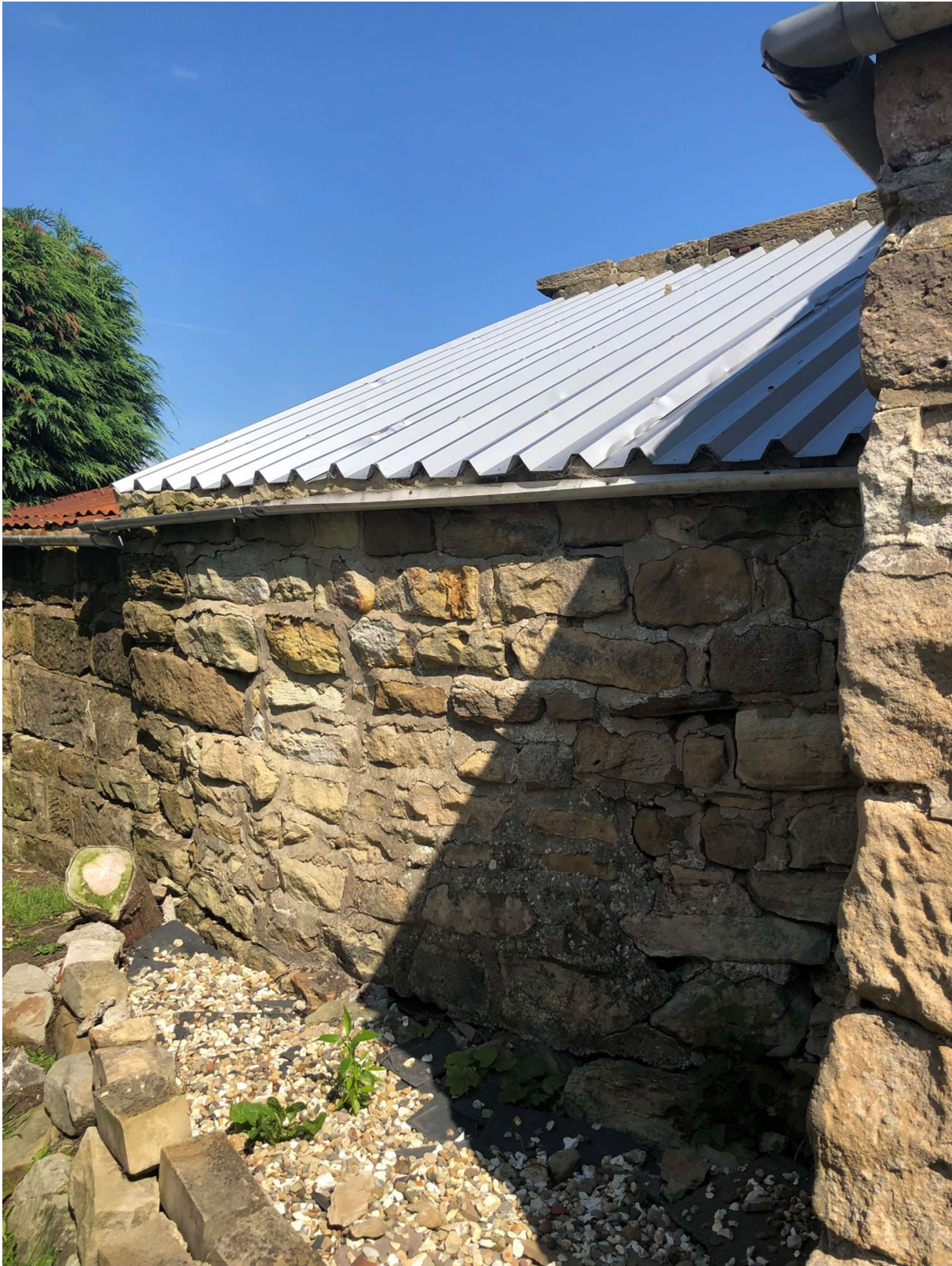
Photograph 4 Side/south of stone lean-to buildings
