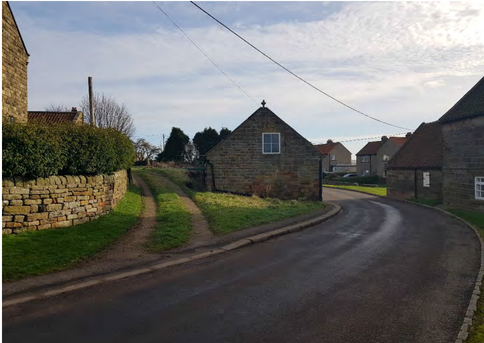
Photo 1 – View of site and access from High Street looking east
