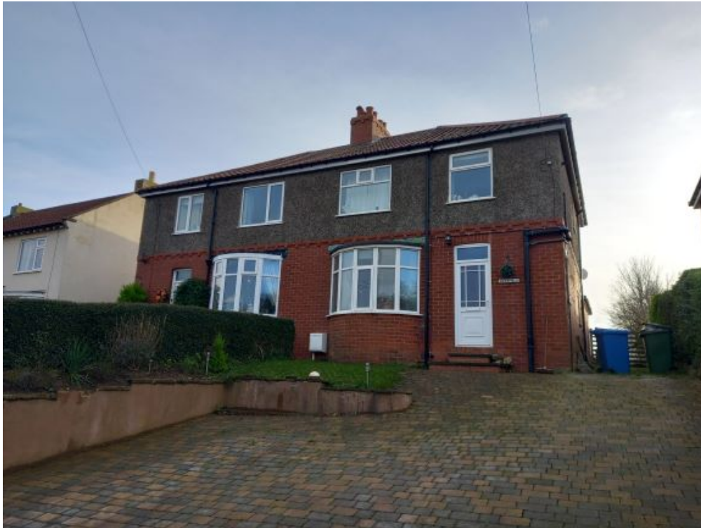
Front elevation of Westfield taken from pavement on Sledgates. It is a two storey, semi-detached property constructed of red brick with pebble-dash render first floor under a hipped roof. The front door is to the right with a large bow window at ground floor to the left.
