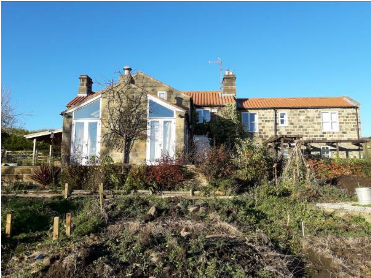
Photo showing existing rear extension at Smoothmans Cottage.
