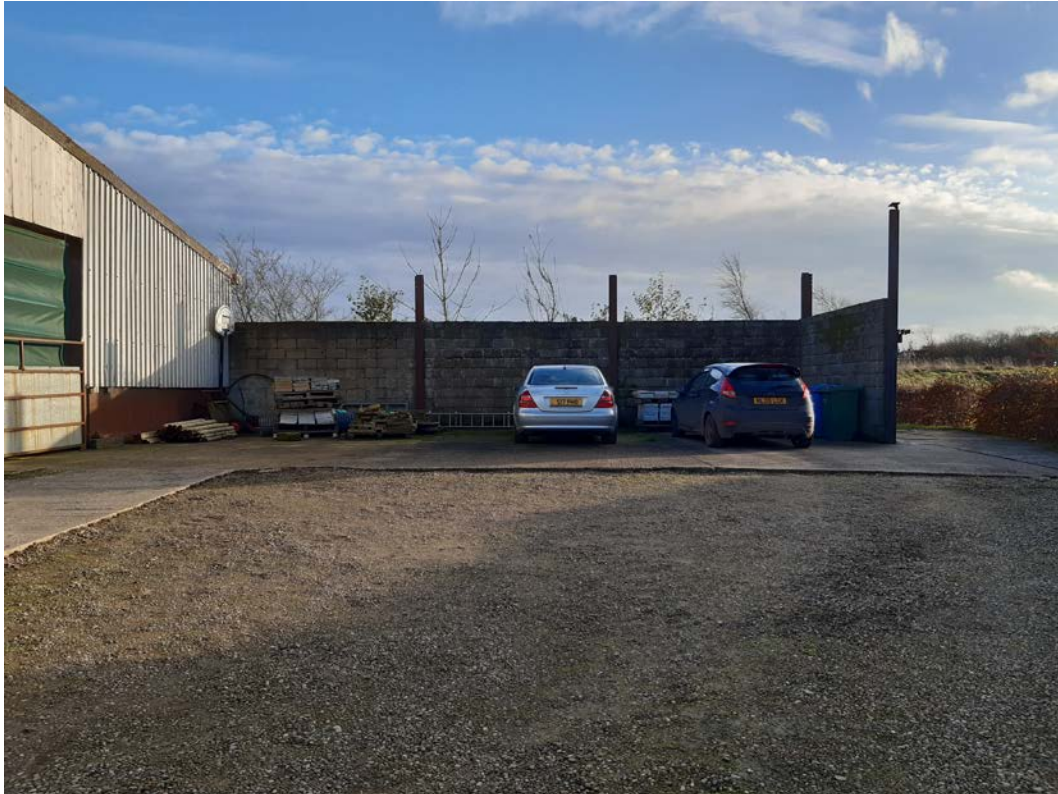
View of the existing concrete hardstanding and concrete block walls which will form part of the proposed garage/workshop/store
