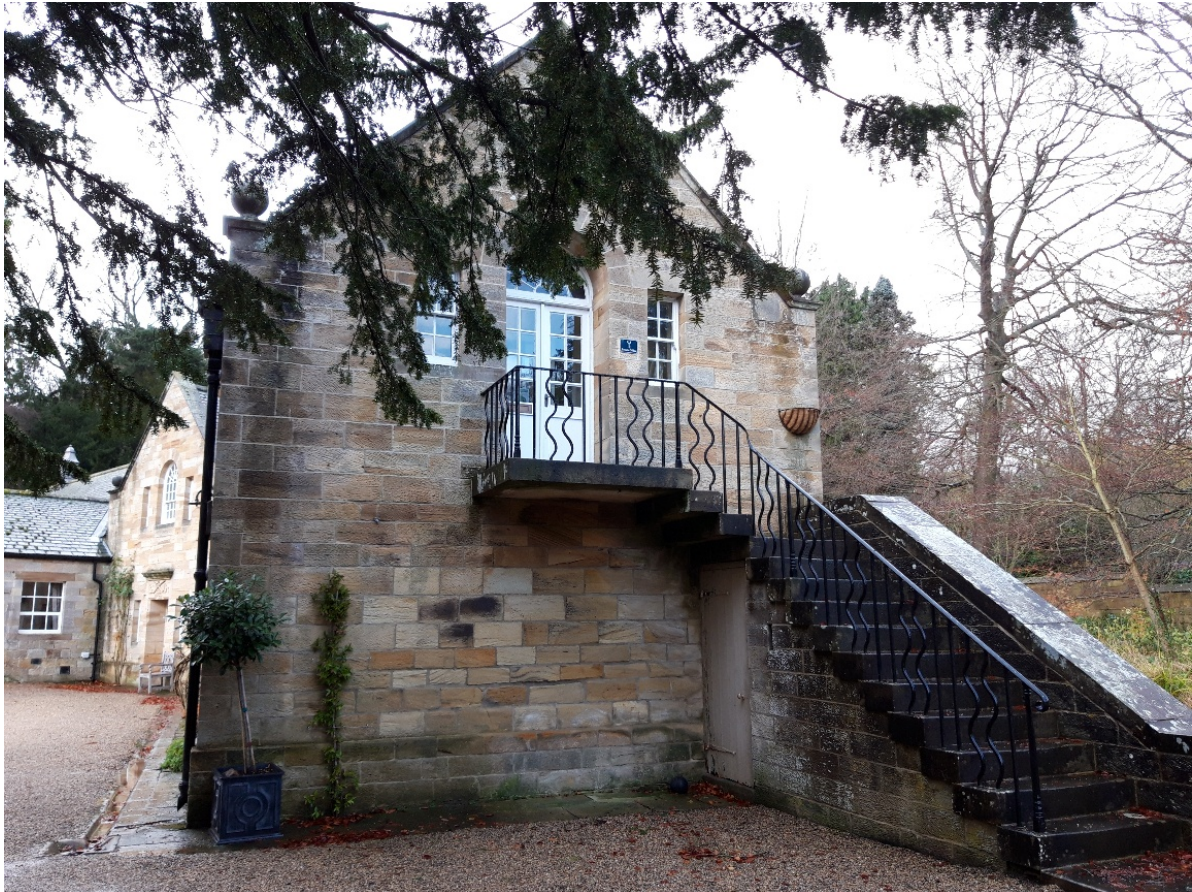
This photo shows the eastern elevation of the outbuilding, including the external staircase under which the extraction unit is to be installed.
