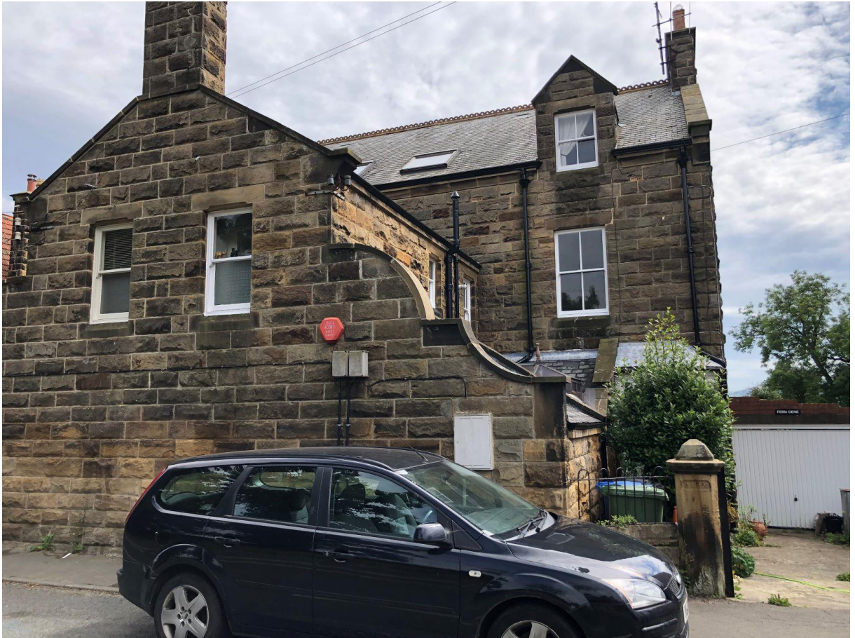
Photograph 2 North west (rear) elevation abutting the Highway
