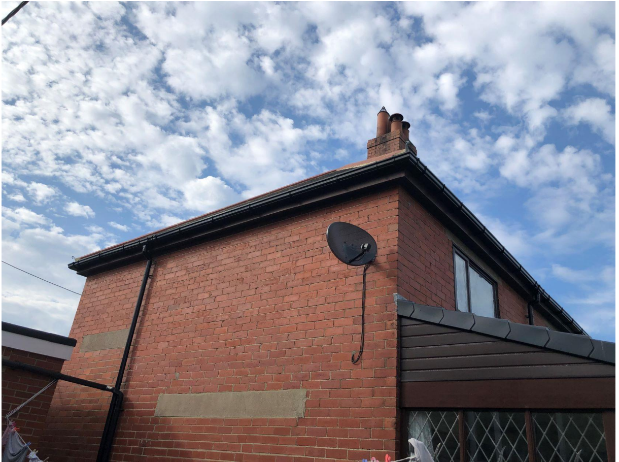
Photograph 3 Side (south) Elevation
