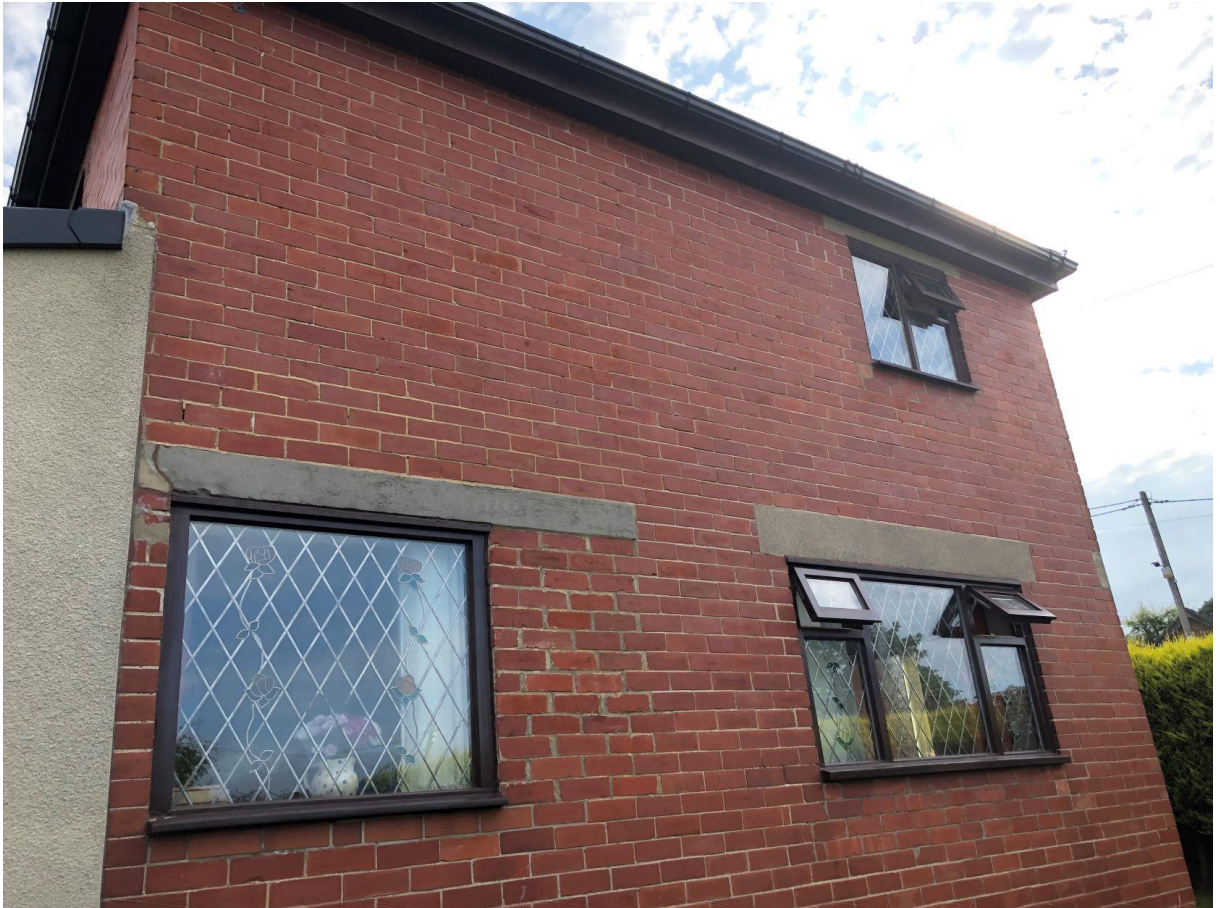
Photograph 4 Side (north) Elevation
