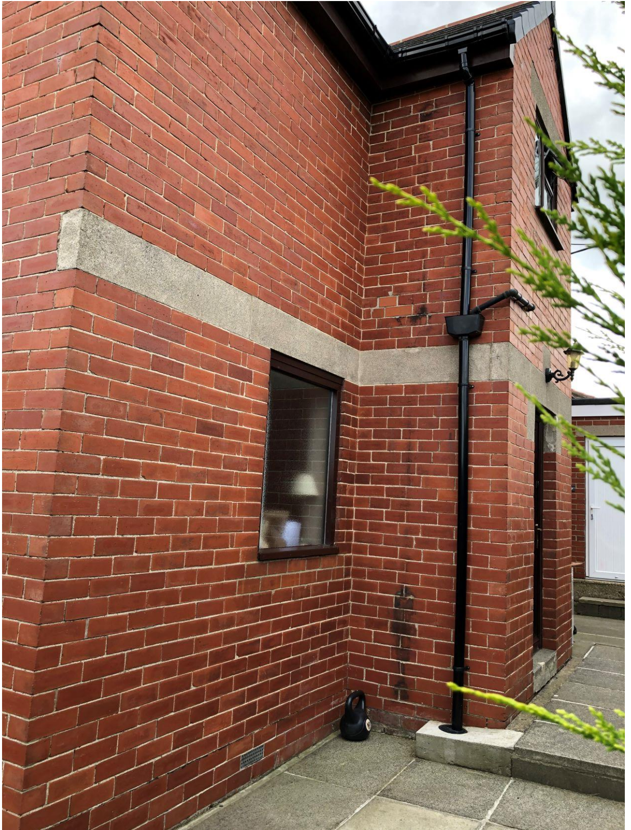
Photograph 1 Part front elevation
