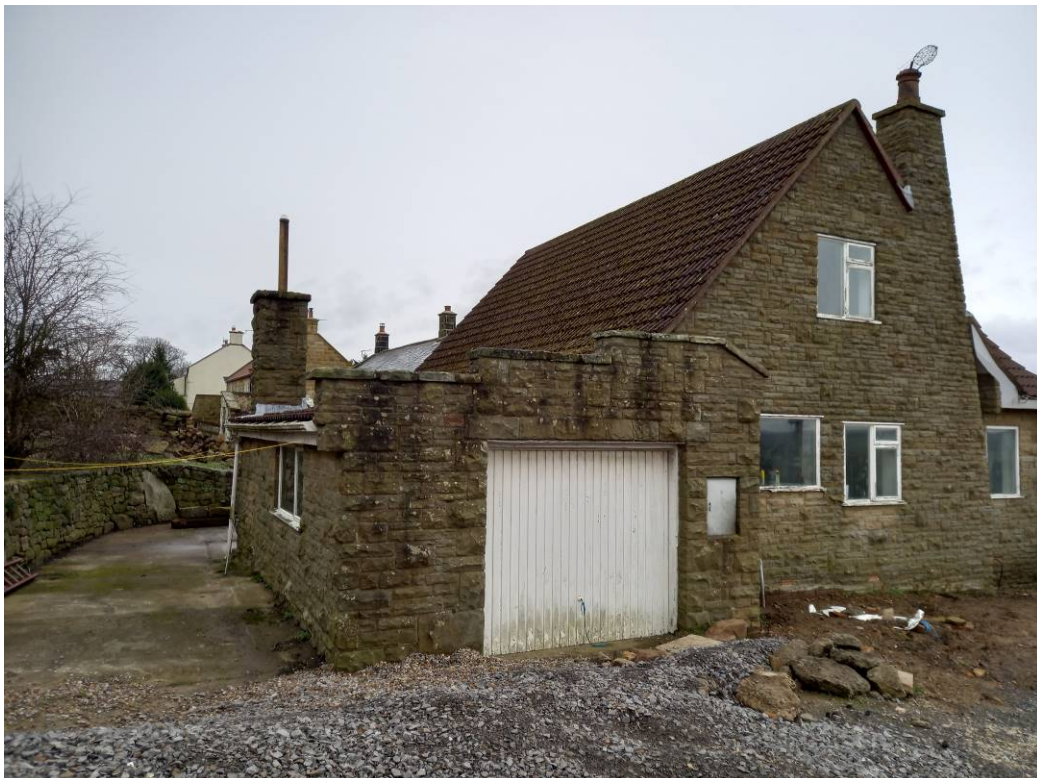
Photograph showing side elevation of Long View, the garage to be demolished and the siting of the rear single storey extension
