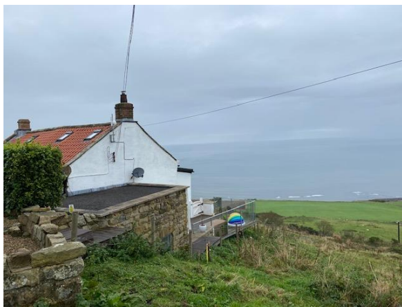
P4, - South side elevation showing the flat roof structure now in situ
