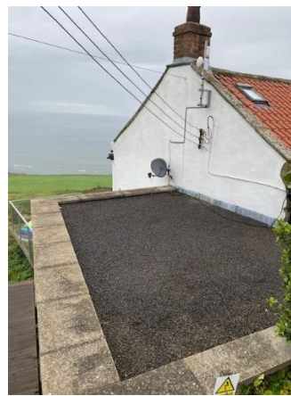
P5, - Flat roof (south side).
