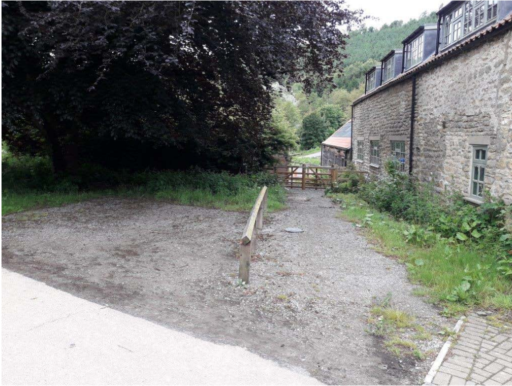
View from the access road to The Bike Barn showing the extensive landscaping about the site screening the container
