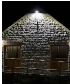
Shielded warm white lights with appropriate controls provide directed light only where and when it is needed.
