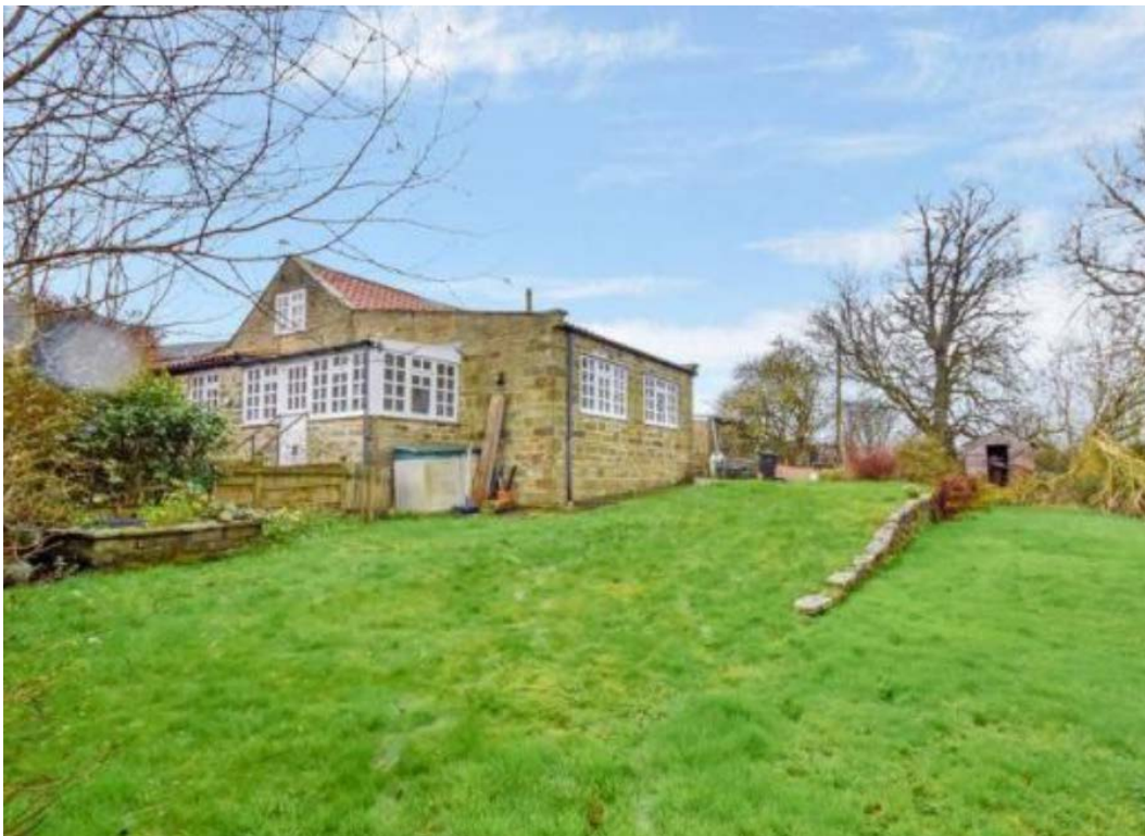
View from east of sunroom to be replaced with pantiled extension incorporating a flue
