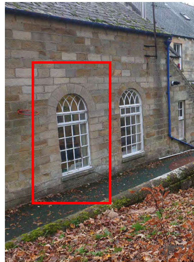
Window to be replaced with a door
