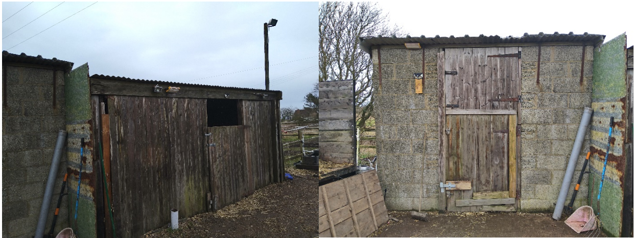
Pictures showing existing stable block.
