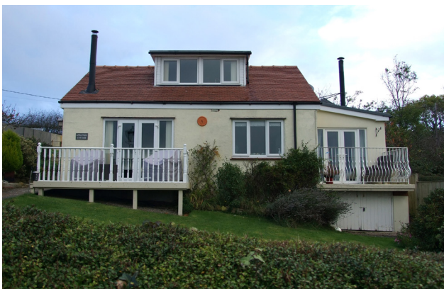
Appletree Cottage primary elevation photographed from the south
