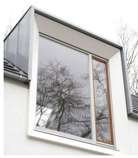
Zinc clad dormer window
