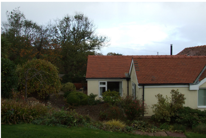
Appletree Cottage side elevation photographed from the west
