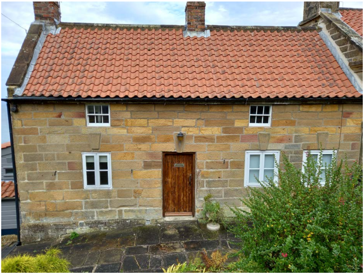
Photograph showing the front (west) elevation of Brow Hill Cottage, Ravenscar
