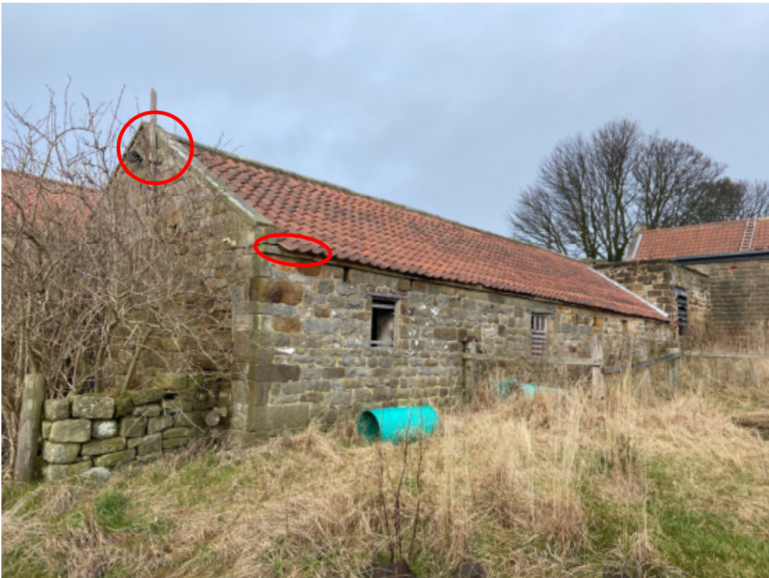
Photo 6. Building 3 – south and eastern elevations. PRFs circled red.
