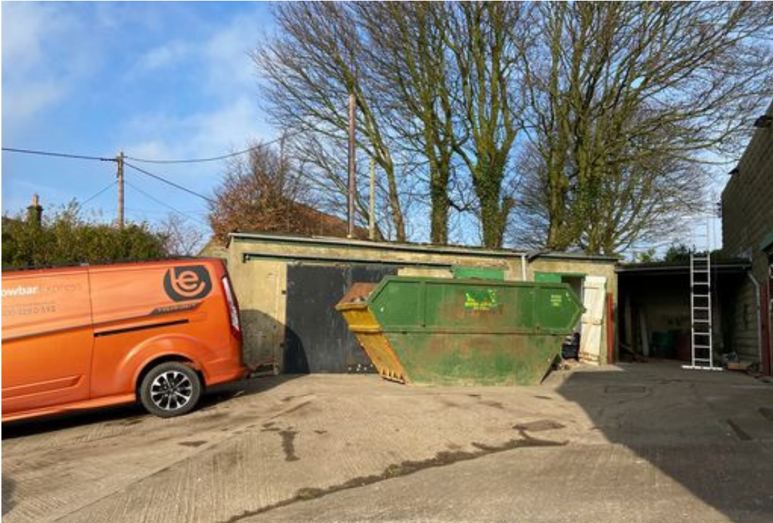
Photo 5. Building 2 – southern elevation.
