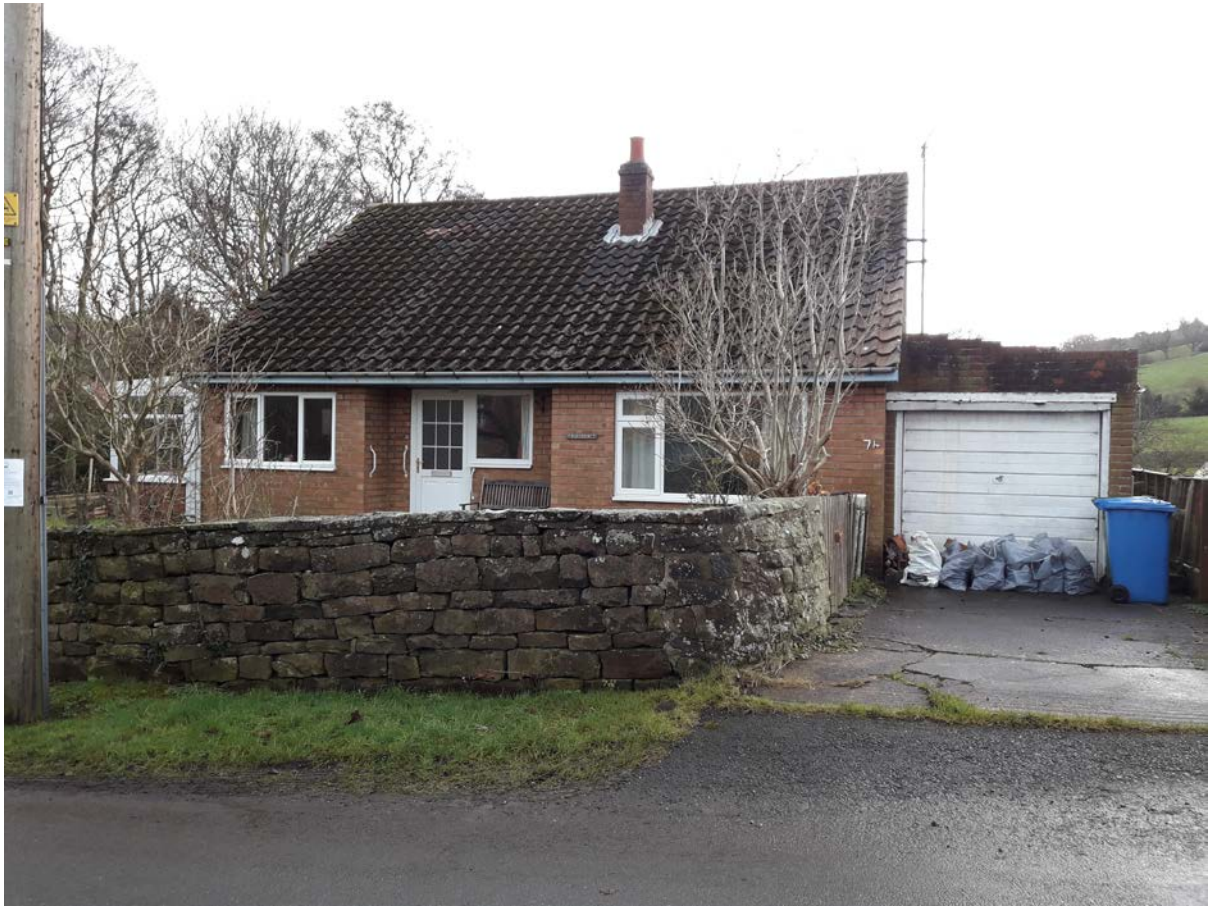
Photo showing front elevation of 74 Iburndale Lane, Sleights.
