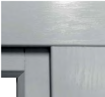
Windows with welded corners (above) are not usually allowed in conservation areas whereas windows with mechanical joints (below) have been approved.
