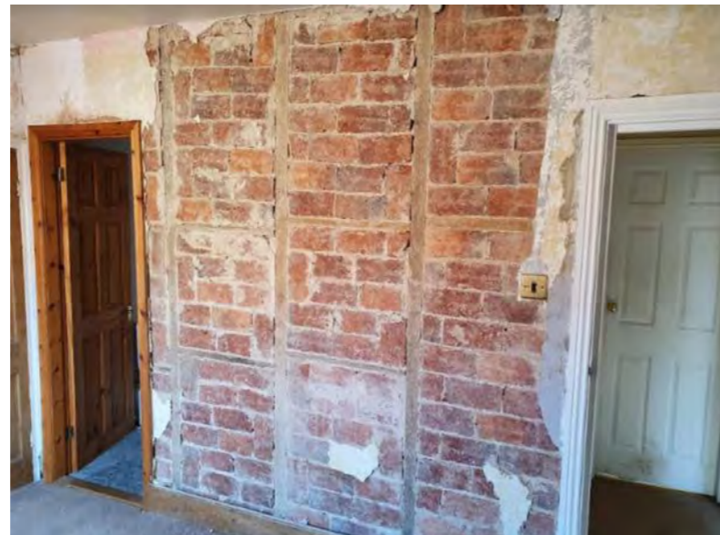
Historic stock brick wall to be finished in quicklime plaster
