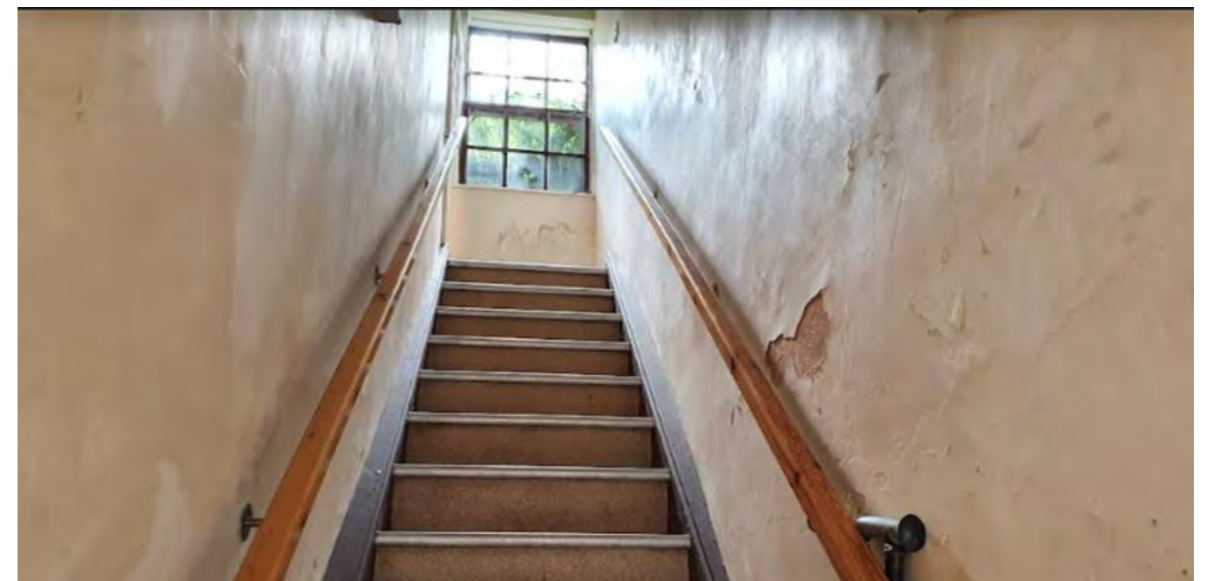
Main staircase to be re-plastered in hotlime
