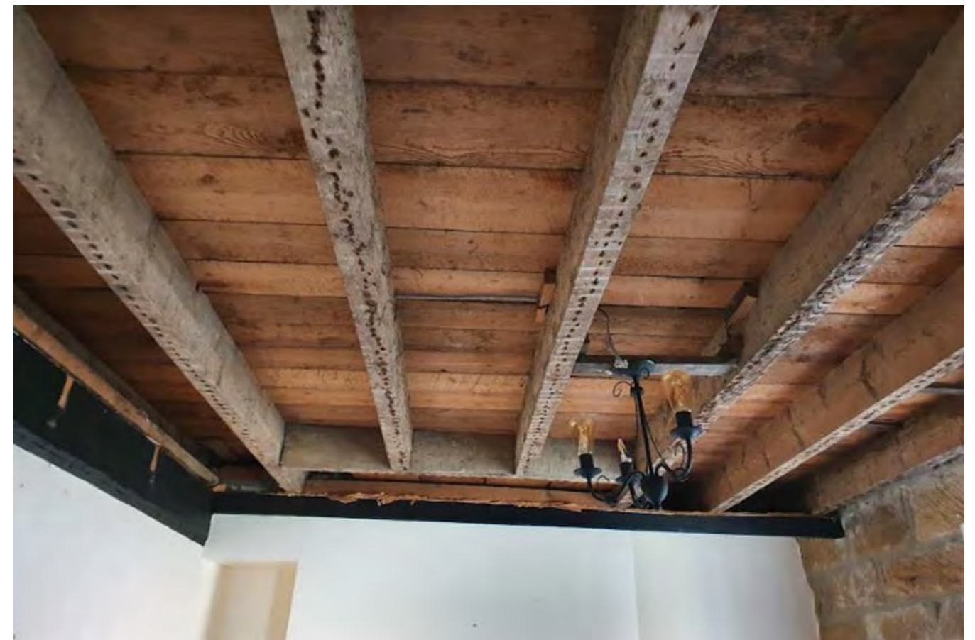
Current missing ceiling and sample of remains of former chipboard ceiling
