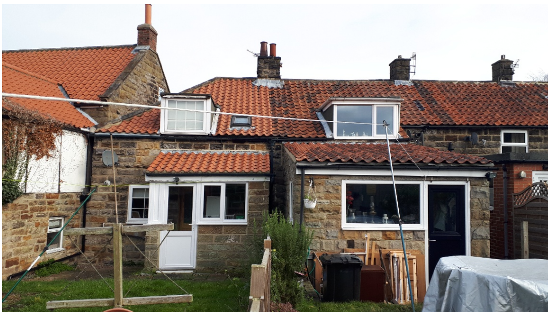
View of the rear of 186 (left) and 184 Coach Road (right). The neighbouring property 186 also has a smaller single storey lean-to extension, and similar dormer.
