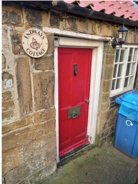
This photo shows the rear door on the north elevation of Endways, Robin Hood's bay.
