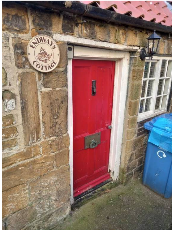
This photo shows the rear door on the north elevation of Endways, Robin Hood's bay.
