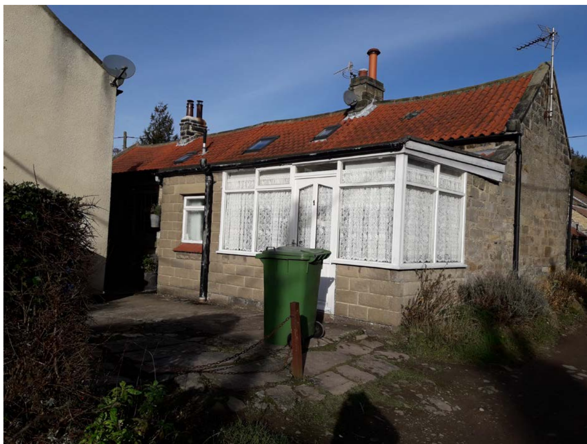
Photo showing rear elevation of Rosedale Cottage and existing extension.
