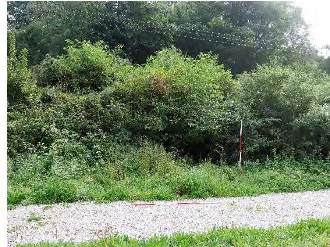
Figure 5: The overgrown earthen bank facing southeast.
