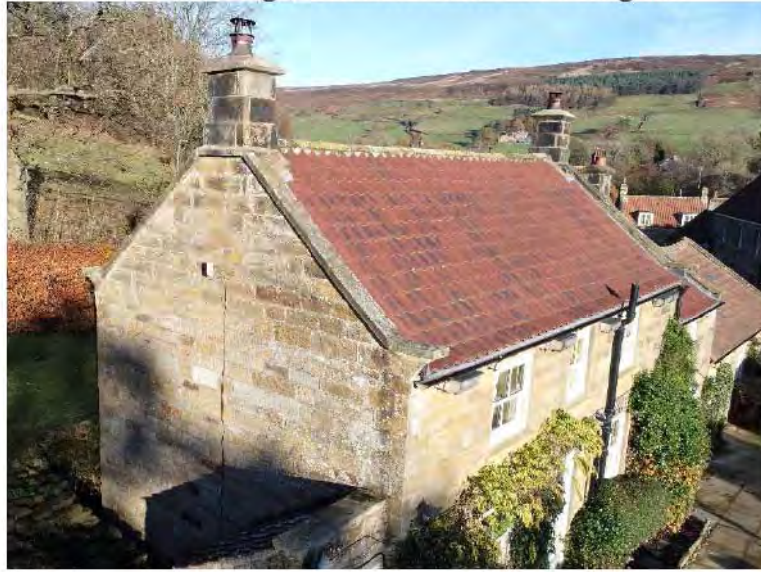
Plate 2 – cottage, north elevation.
