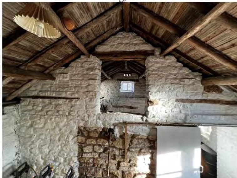
Plate 6 – outbuilding, internal roof void.
