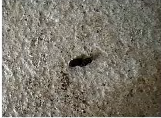
Plate 7 – bat dropping located inside the outbuilding.
