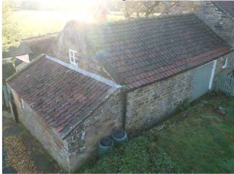
Plate 4 – outbuilding, north elevation.
