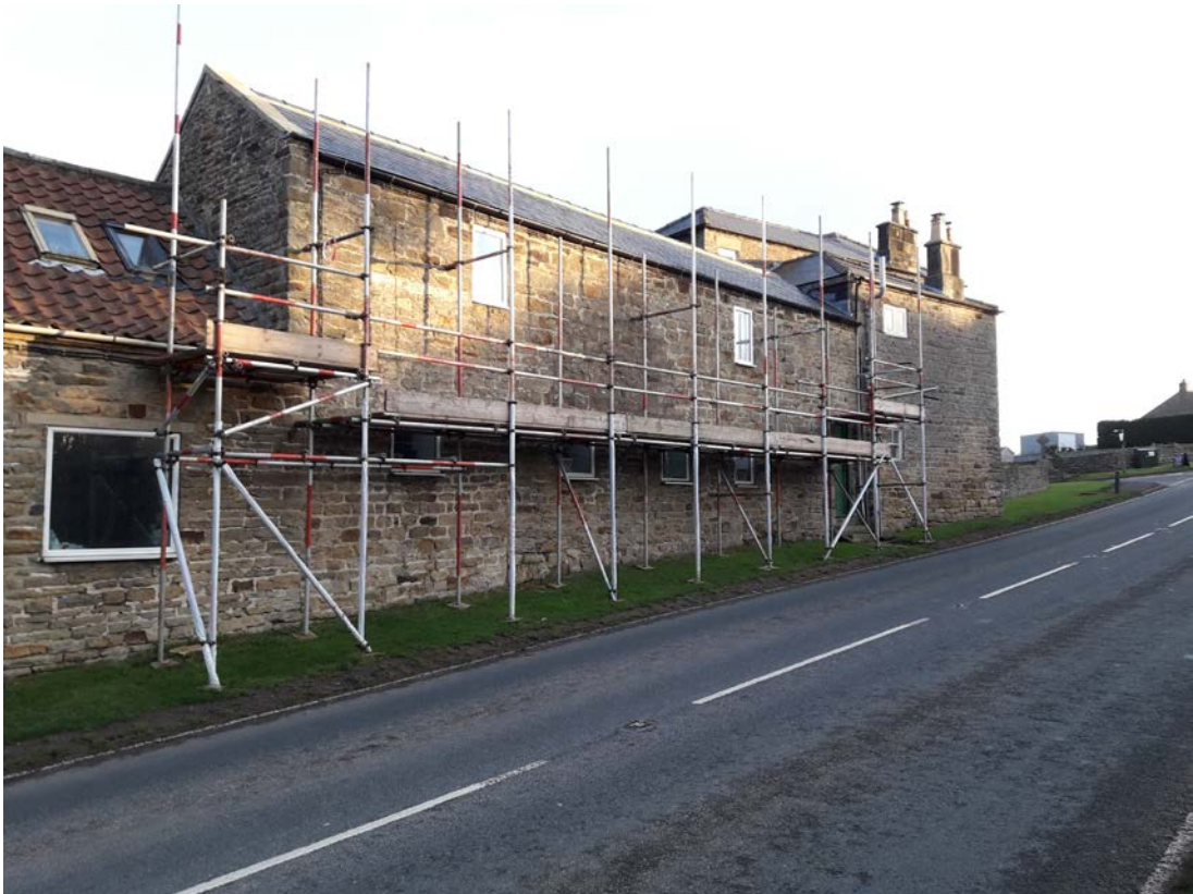
Photo showing front elevation of The Cottage, Sneaton Hall, Sneaton.
