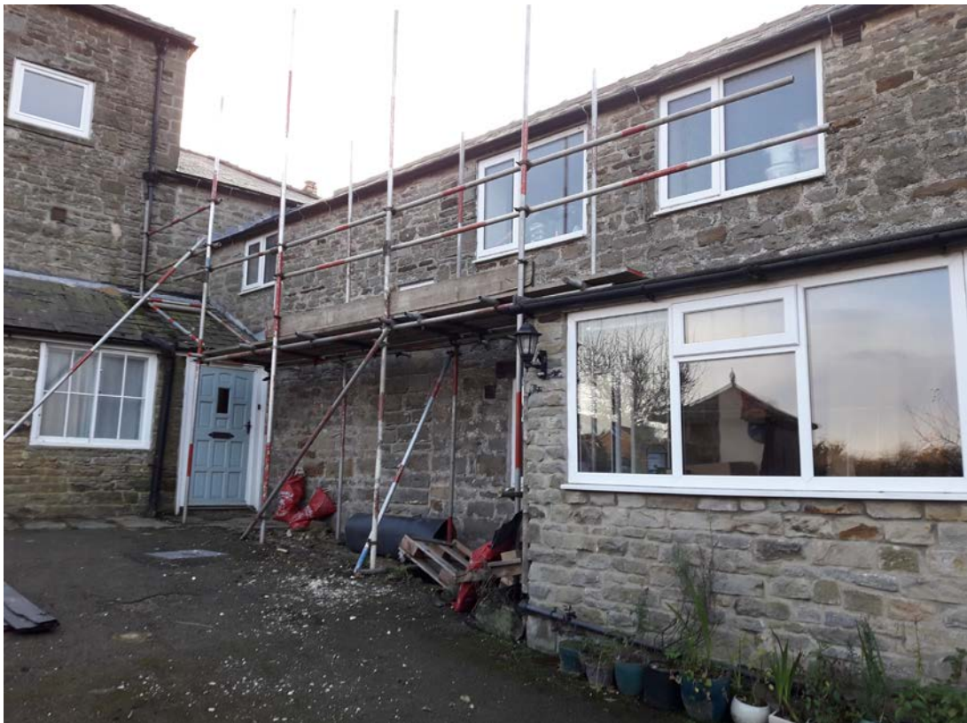
Photo showing the rear elevation of The Cottage, Sneaton Hall, Sneaton.
