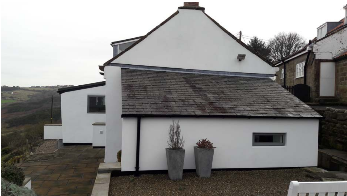
Side elevation of Susanna Hill Cottage showing the existing dining room extension and front lean-to projection
