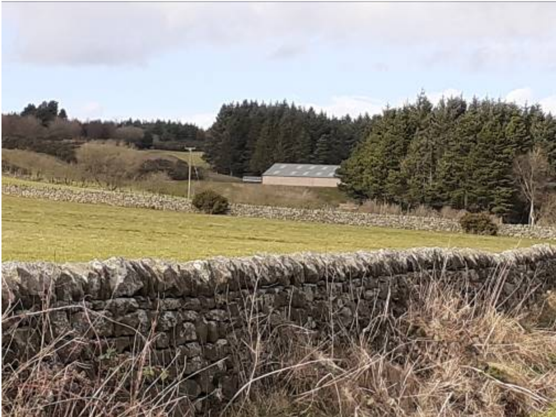
Zoomed in photo of existing building – extension to the rear
